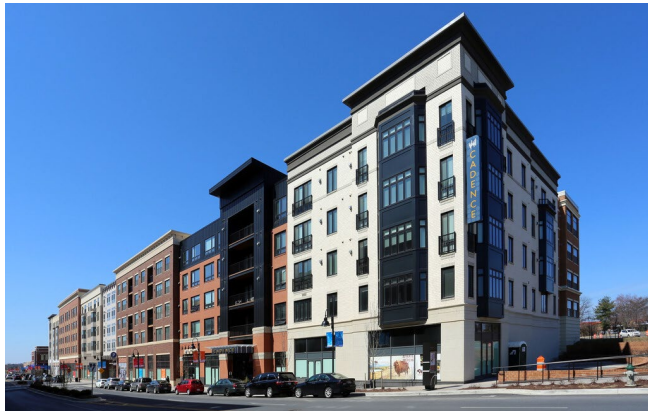
83% of SF is Multifamily-Anchored: 113 Ellington Blvd., Rockville (Cadence at Crown)
