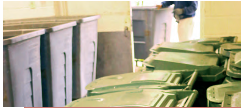
Trash room/loading dock area where recycling and refuse are picked up by the collector
