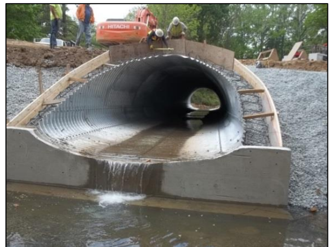
Hillendale Road Storm Culvert Replacement Project
