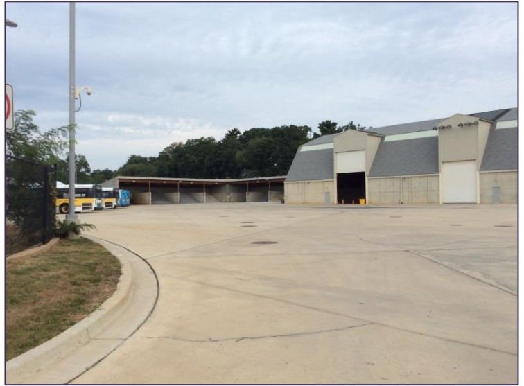
Salt Storage Barn at new Highway Services Depot
