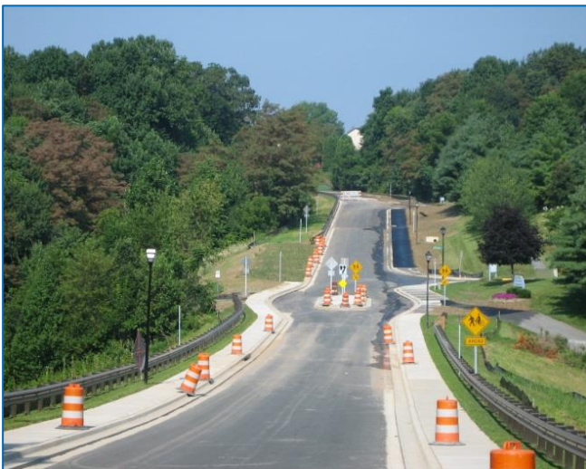
Valley Park Drive road extension project in North Bethesda
