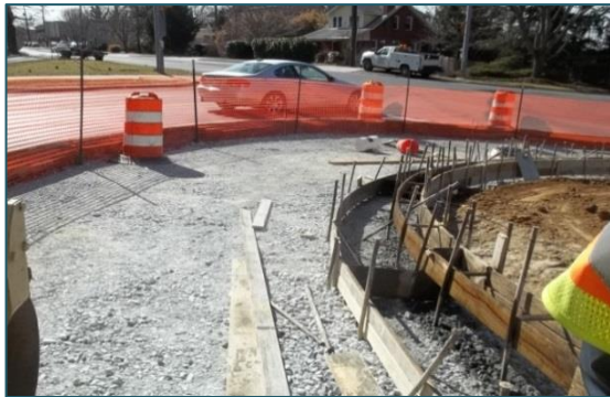
Concrete Curb and Sidewalk added to an intersection in Olney
