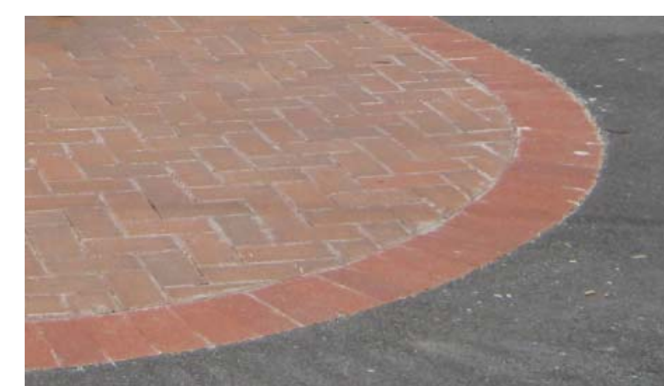
Brick Pavers with Existing Asphalt Trail
