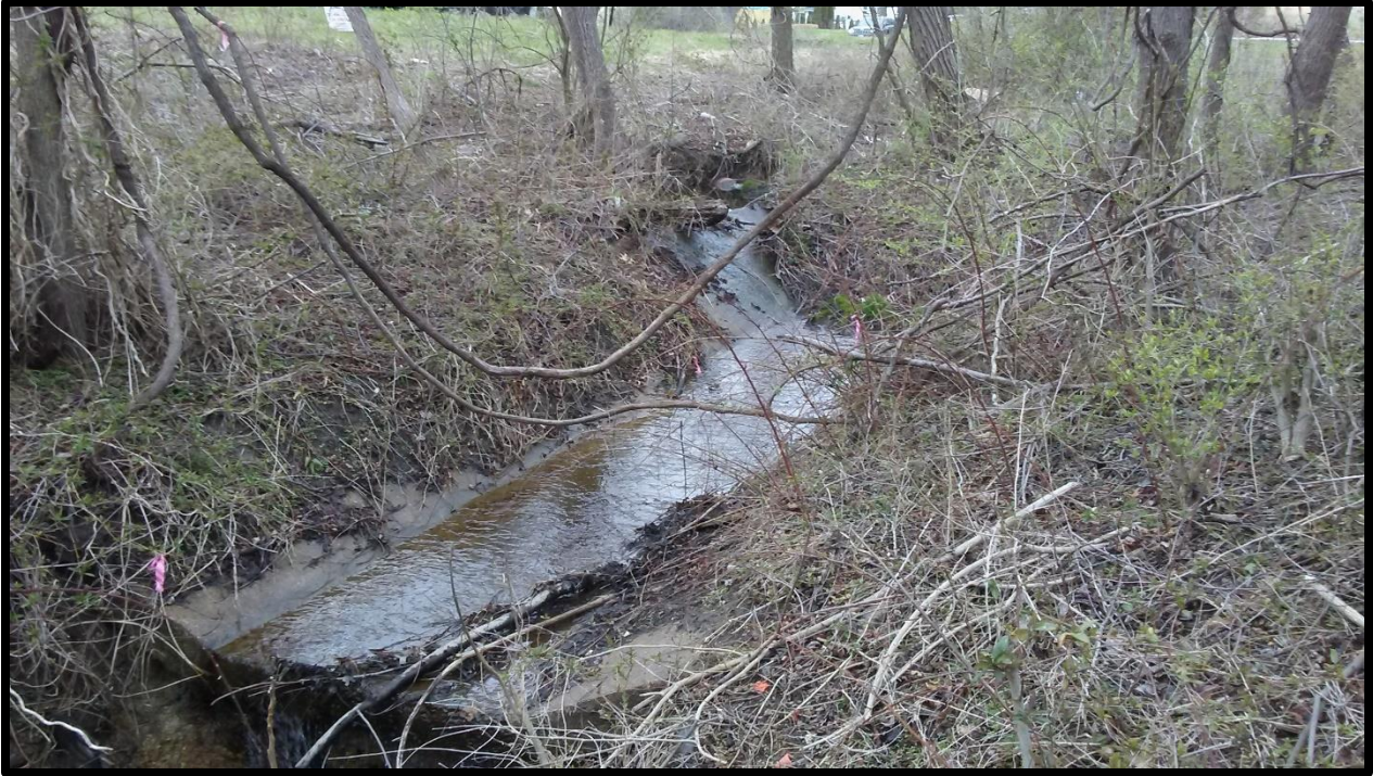
Figure 16. Concrete-lined stormwater outfall extending from under the MD 355/MD 121 intersection. View looking to the north.
