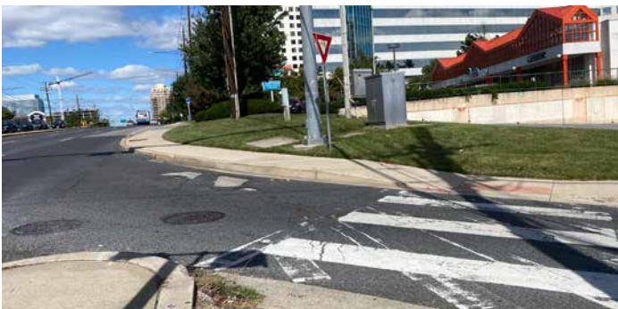
Right-Turn Slip Lane and Sidewalk at Nicholson Lane & Rockville Pike
