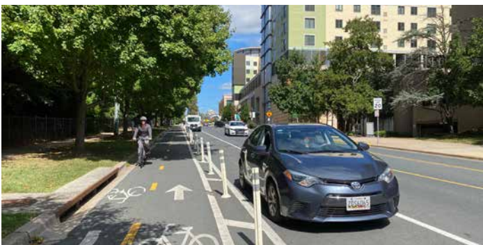
Two-Way Separated Bike Lanes along Woodglenn Drive
