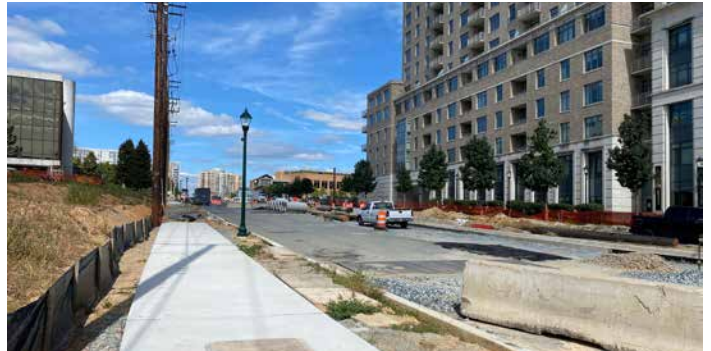
Shared Use Path along Towne Road/Hoya Street
