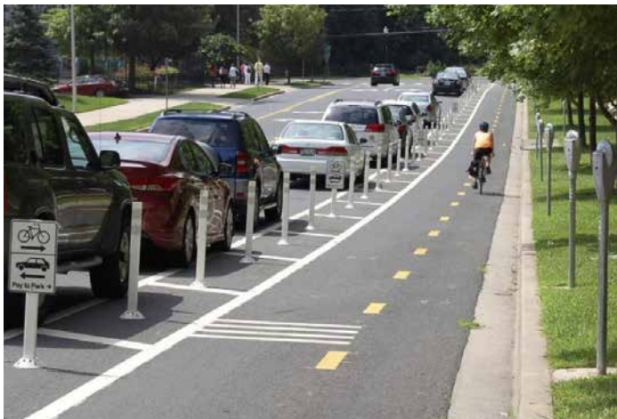
Two-way Separated Bike Lanes extending the BTT along Woodglan Drive to Nicholson Lane. Source: Montgomery County Planning Department
