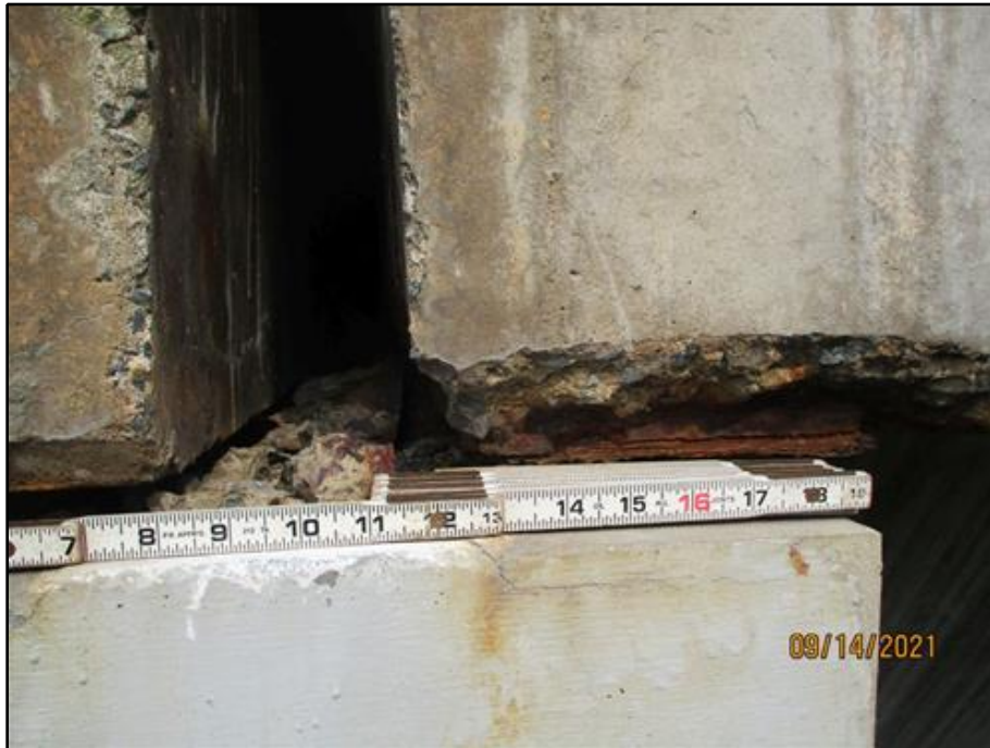
37. Corner spall on the west end of Beam 1 in Span 14 at Buttress 27
