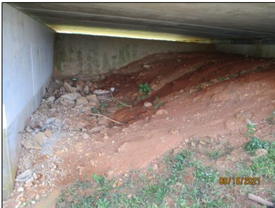
42. Loose soil and rocks in front of the north end of the west abutment
