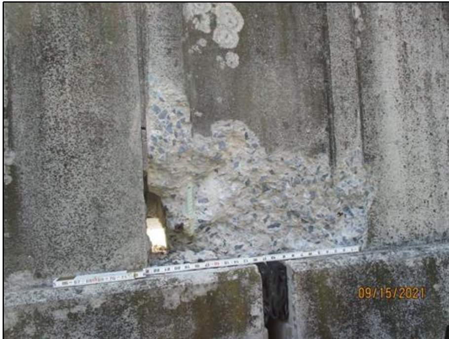
11. Full depth spall with exposed epoxy coated steel reinforcing in the exterior face of the north parapet above Buttress 3
