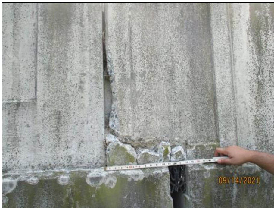
13. Spalling in the north face at the base of the north parapet over Butress 27
