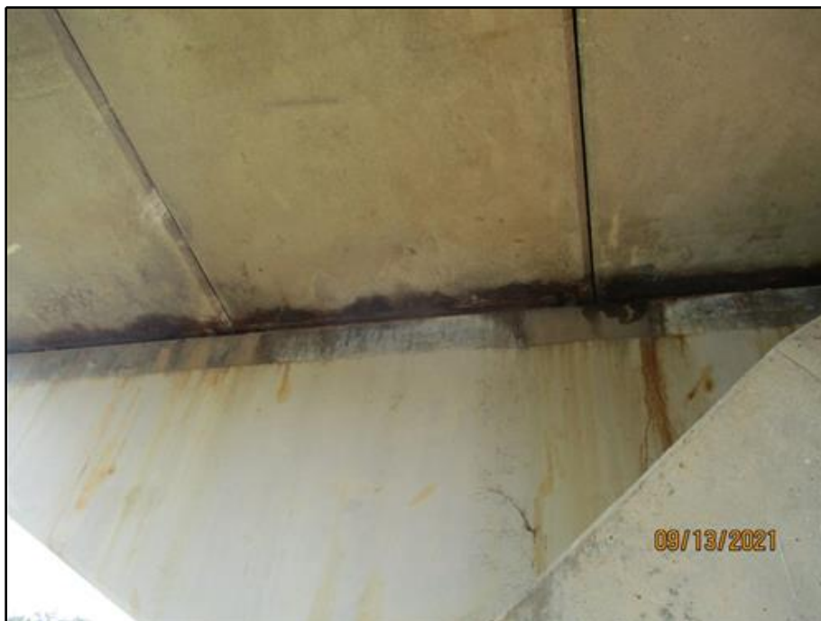
26. Typical active water leakage between beams (Beams 2 and 3 at west face of Buttress 3)
