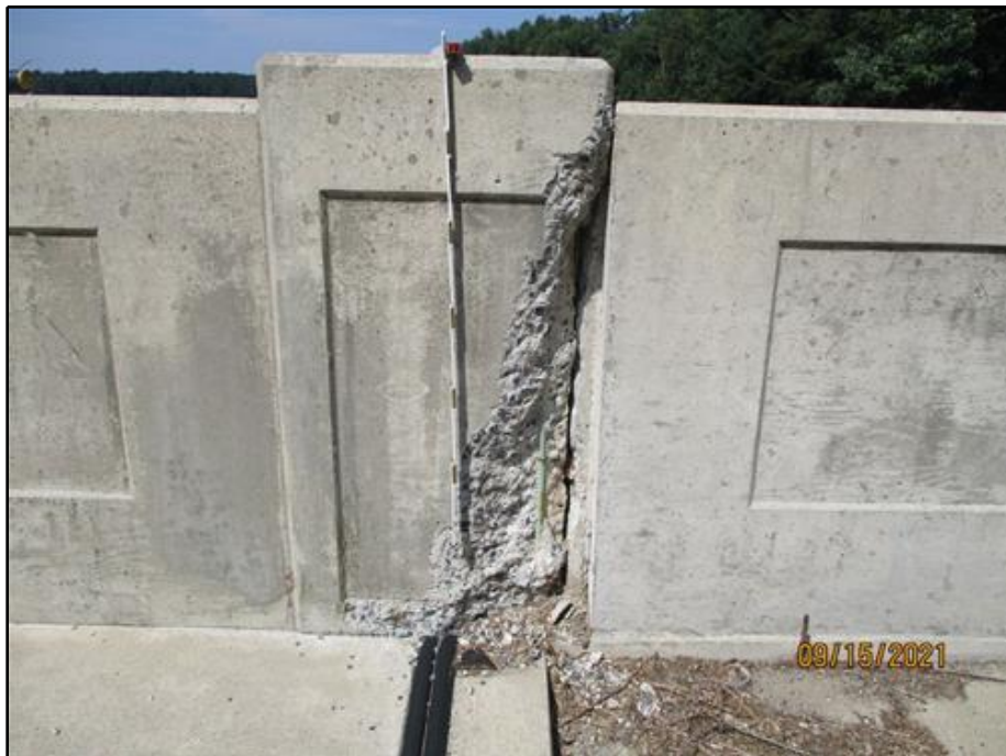
10. Spall in the south face of the north parapet above the east abutment
