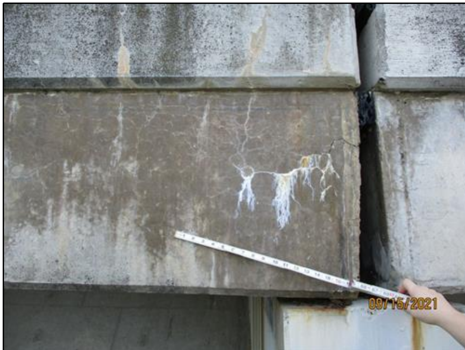
32. Map cracking with efflorescence in the north face of Beam 9 in Span 4 at Buttress 7
