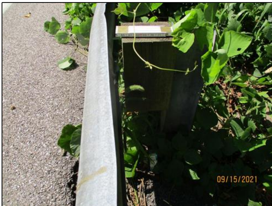
56. Post 17 is detached from the northeast approach traffic barrier
