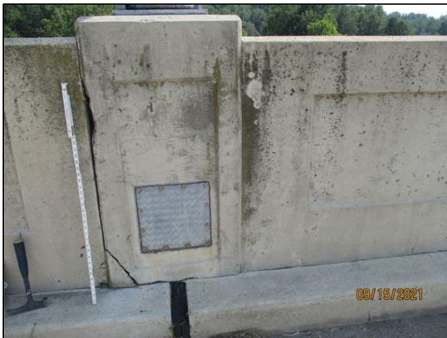
16. Imminent spall in the north face at the base of the south parapet above Buttrass 19
