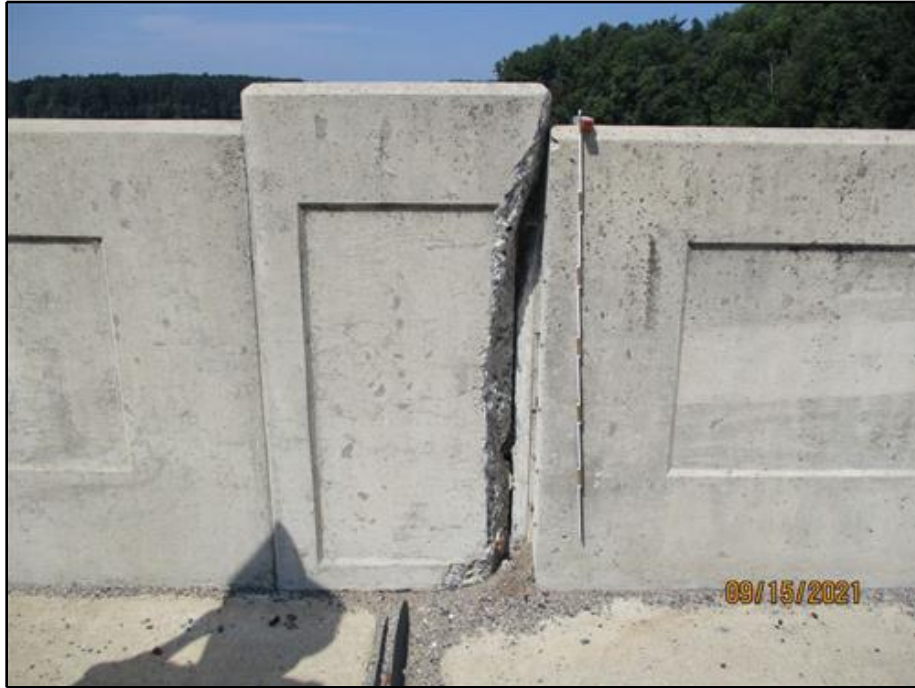
9. Spall on the south face of the north parapet above Buttress 23
