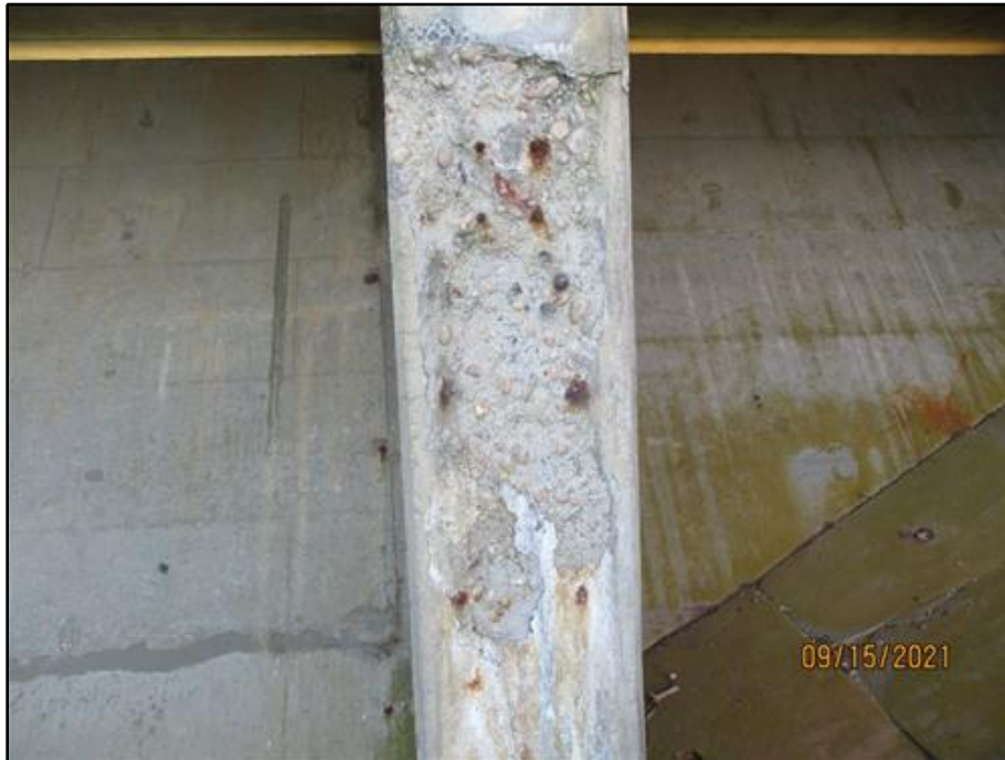
51. Full width spall in the north face of Buttress 3, five feet (5 ft.) below the cap
