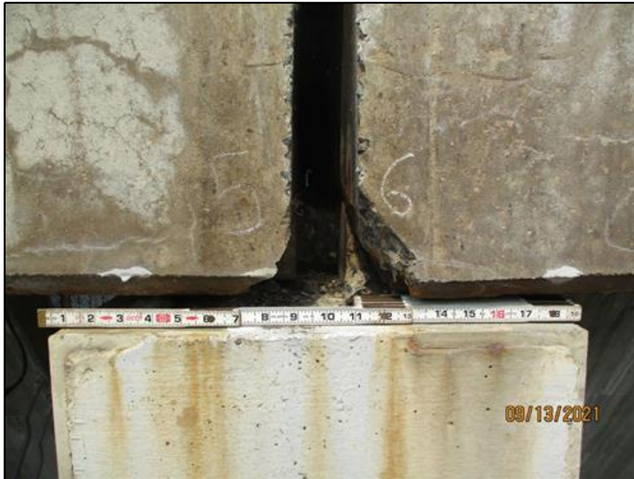
25. Full width spall on Beam 1 at the east end of Span 5 and west end of Span 6 at Buttress 11
