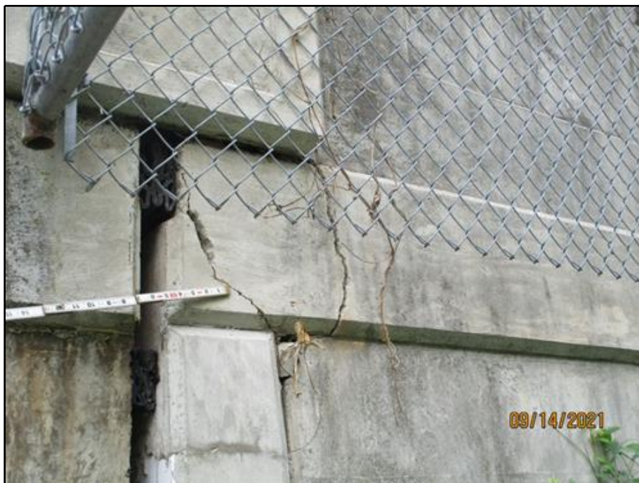
54. Cracks in the south face of the southeast approach traffic barrier at the east abutment
