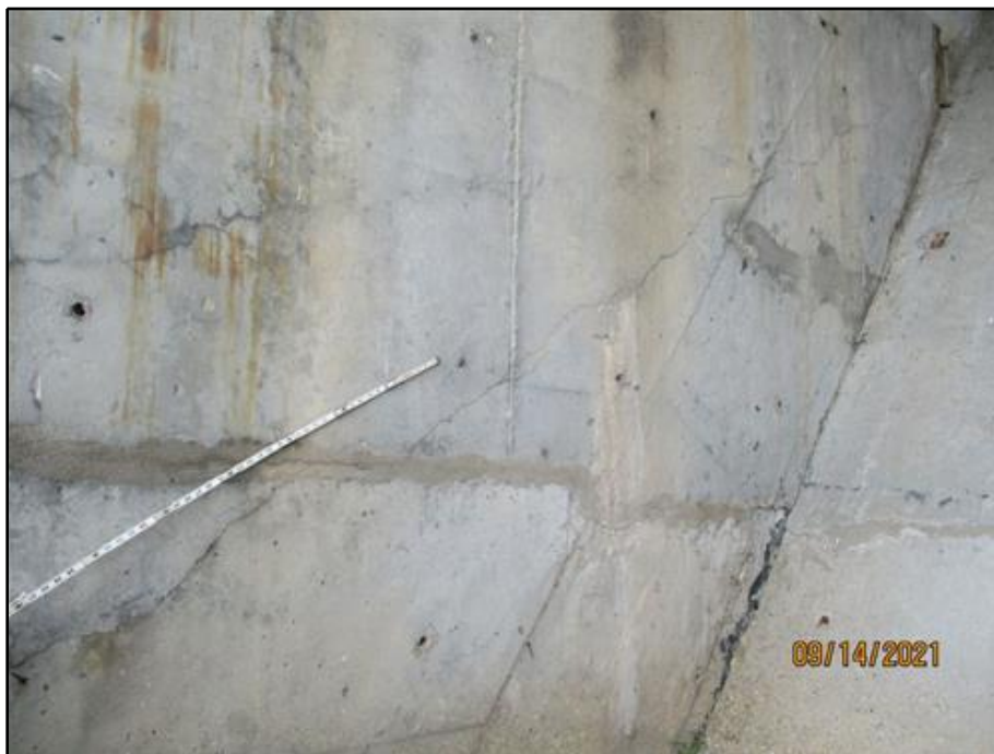
47. Typical diagonal crack in the buttress column along the dam wall (west face of Buttress 27 shown)
