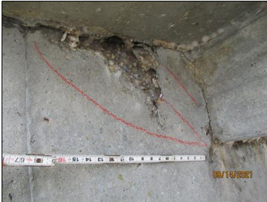
53. Typical spall and delaminated area under the north flange of the walkway (west face of Buttress 25 shown)
