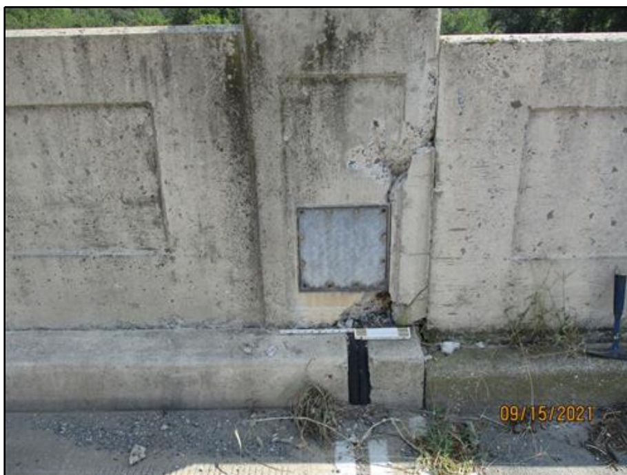
14. Imminent spall in the north face of the south parapet at the west abutment joint
