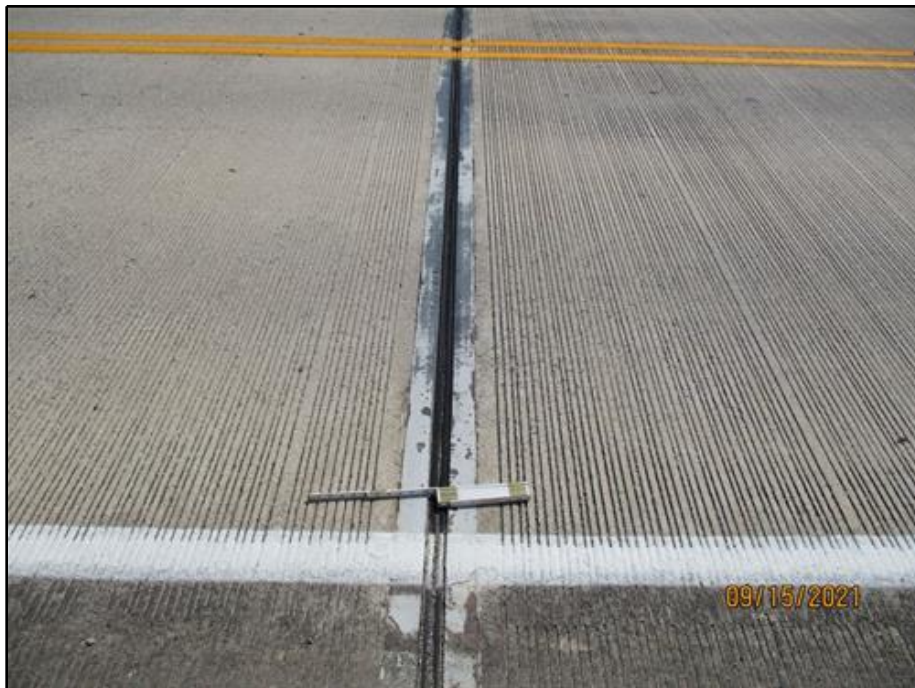
18. Typical compression joint seal condition (Joint 17, looking south shown)
