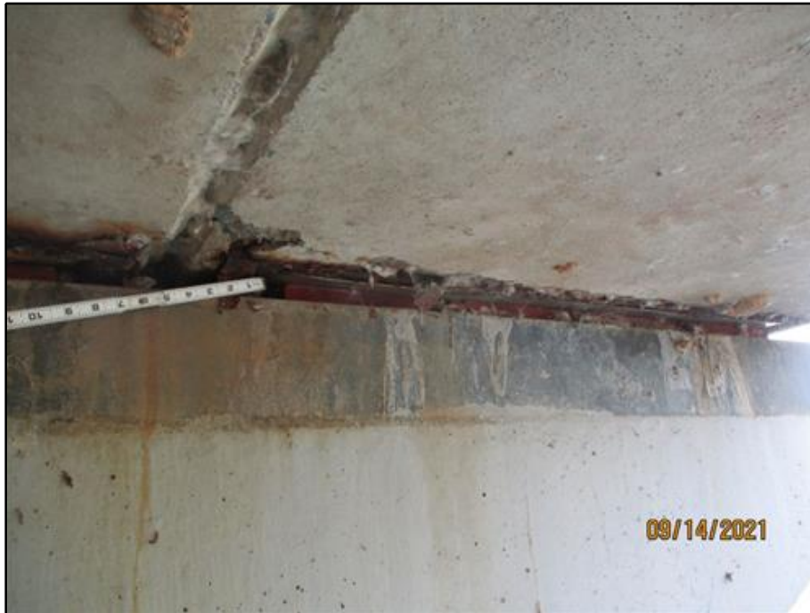
23. Typical delamination at beam corners near bearings (Beam 9 in Span 14 at Buttress 27 shown)
