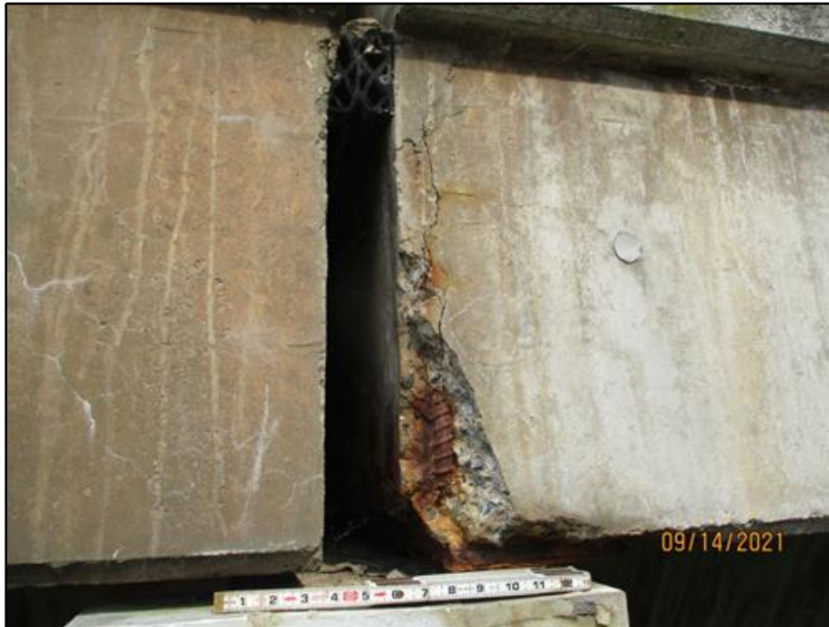
39. Corner spall on the southwest corner of Beam 1 in Span 15 at Buttress 29
