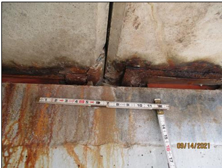
21. Typical exposed and corroded bearing plates (Beams 1 and 2 in Span 13 at Buttress 27 shown)
