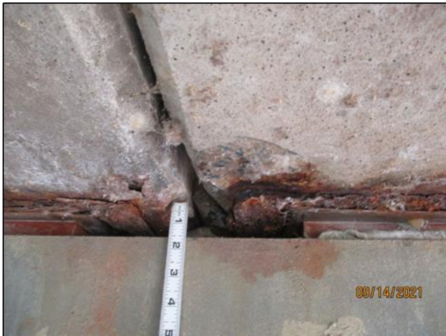
24. Spall with exposed bearing plate at the west end of Beam 2 in Span 6 at Buttress 13
