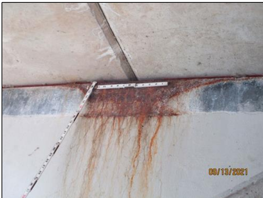
46. Typical moderate corrosion at buttress angles (Buttress 5 between Beams 2 and 3 in Span 3 shown)
