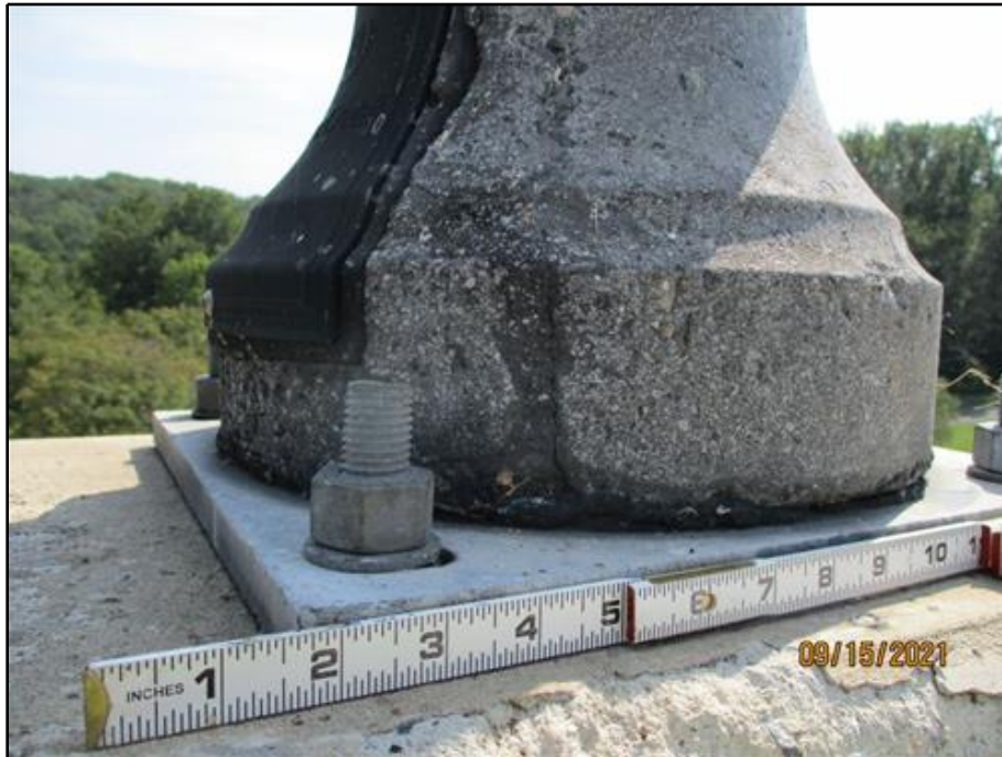
19. Typical crack in the lamp post base (lamp post on the south parapet above Buttress 7 shown)
