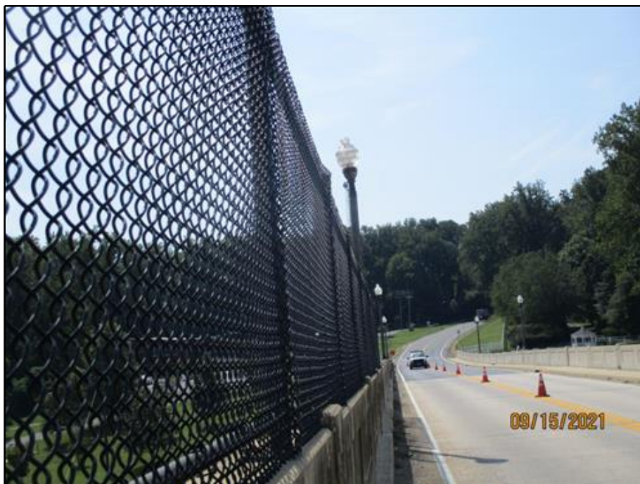
20. Light fixture leaning east relative to the post (lamp post on south parapet above Buttress 7 shown)
