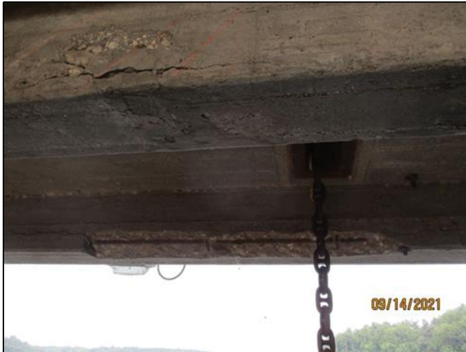
41. Spall with exposed , corroded steel stirrups and abandoned conduit in the south corner of the north stem of the walkway support between Buttresses 24 and 25
