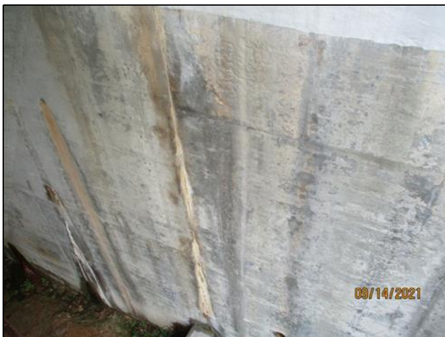
44. Full height crack with efflorescence in the east abutment
