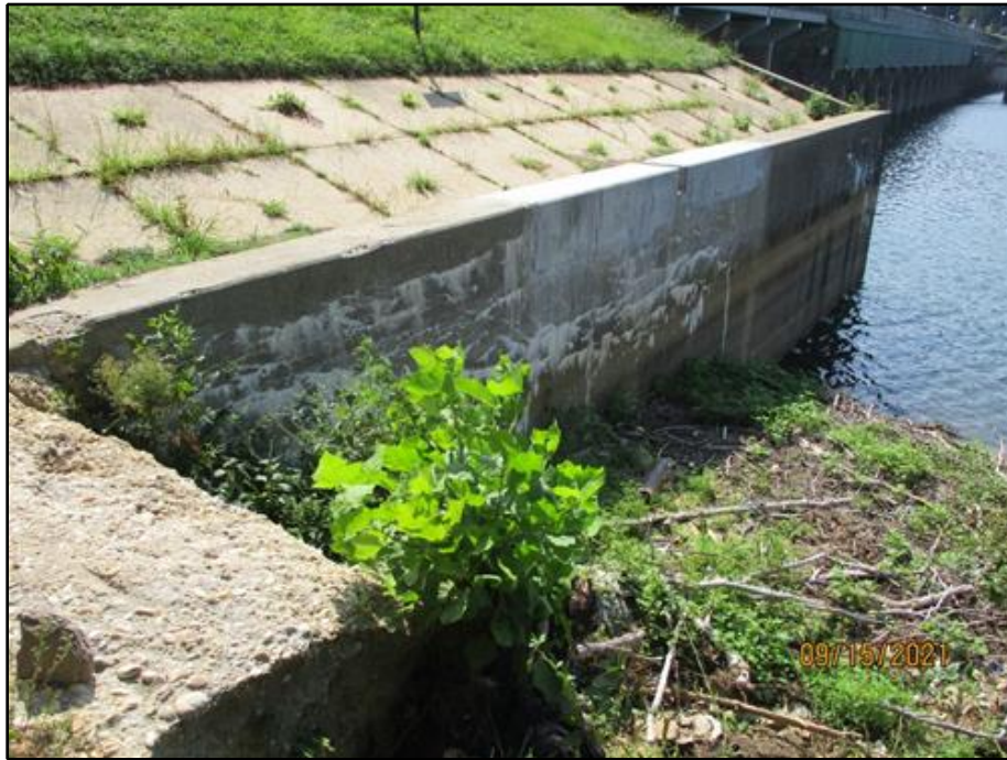
45. Map cracking and efflorescence on the northeast retaining wall. Note the vegetation growing between concrete slope protection panels above the wing wall
