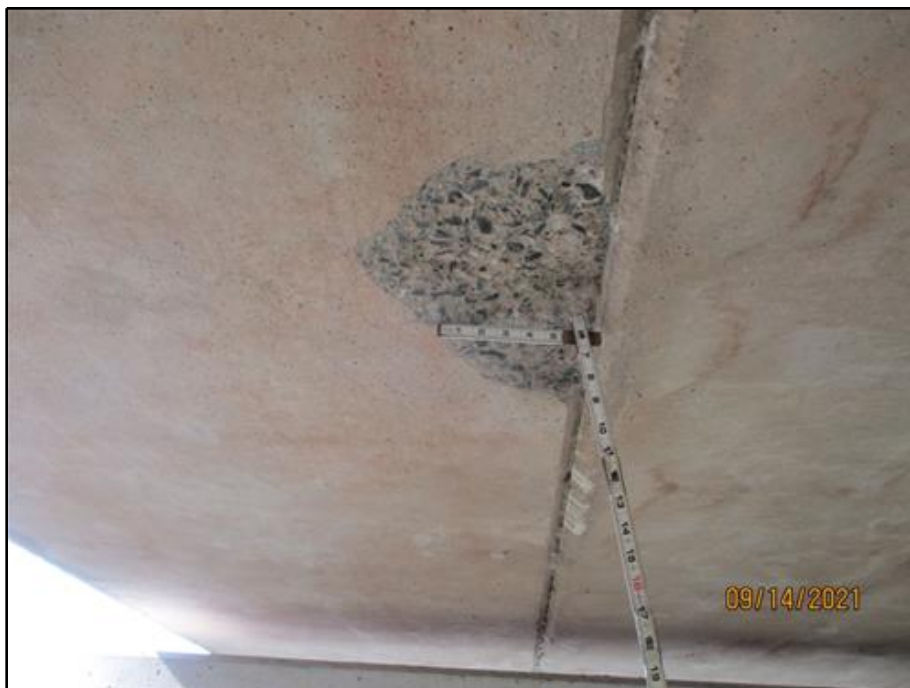
38. Spall in Beam 1 at Joint 1 in Span 14, four feet (4 ft.) east of Buttress 28
