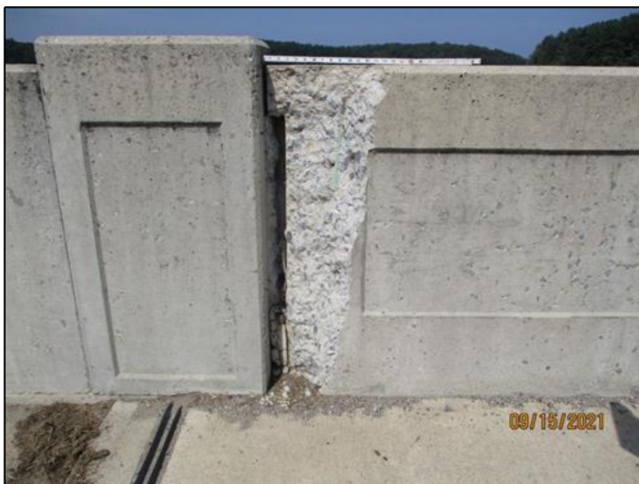
8. Spall with exposed steel reinforcing on the south face of the north parapet at the west abutment
