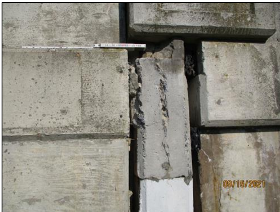
43. Delaminated area and spalls in the south face of the west abutment backwall
