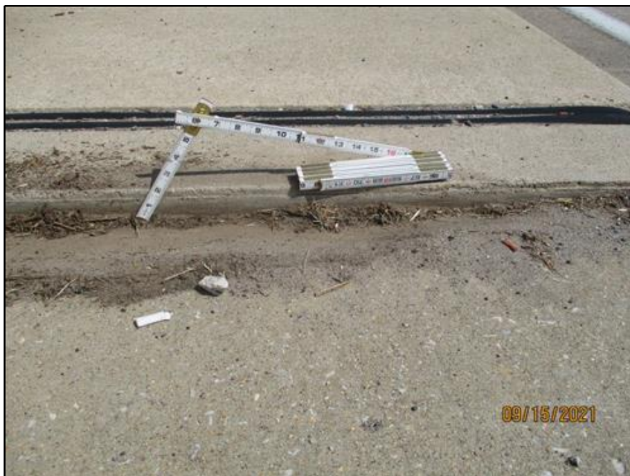
58. Typical settlement of the sidewalk at the approach transitions (northwest approach sidewalk transition shown)
