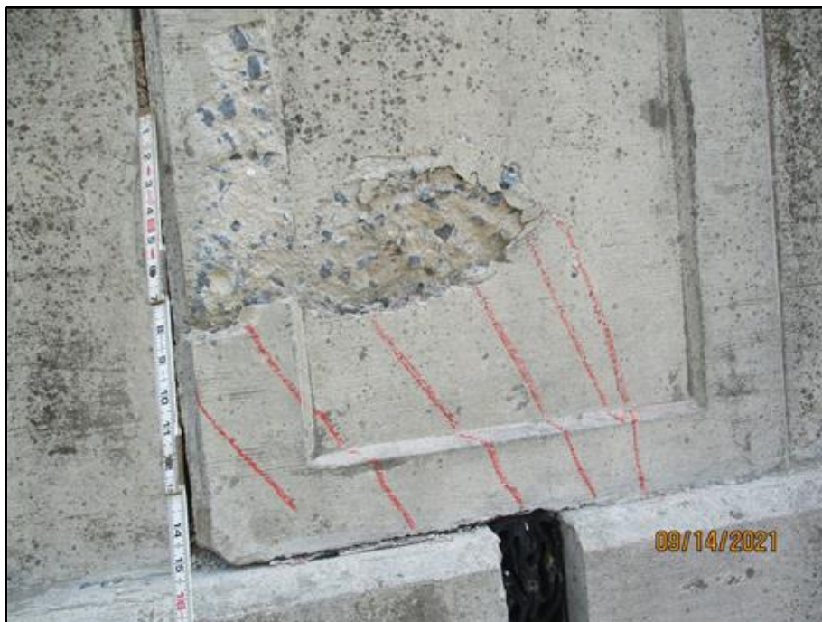
12. Delaminated area on the north face of the base of the exterior face of the north parapet above Buttress 11
