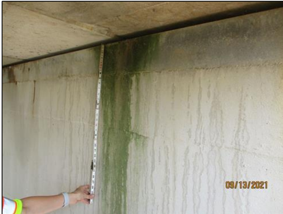
27. Typical active water leakage between beams (Beams 1 and 2 at west face of Buttress 13 shown)
