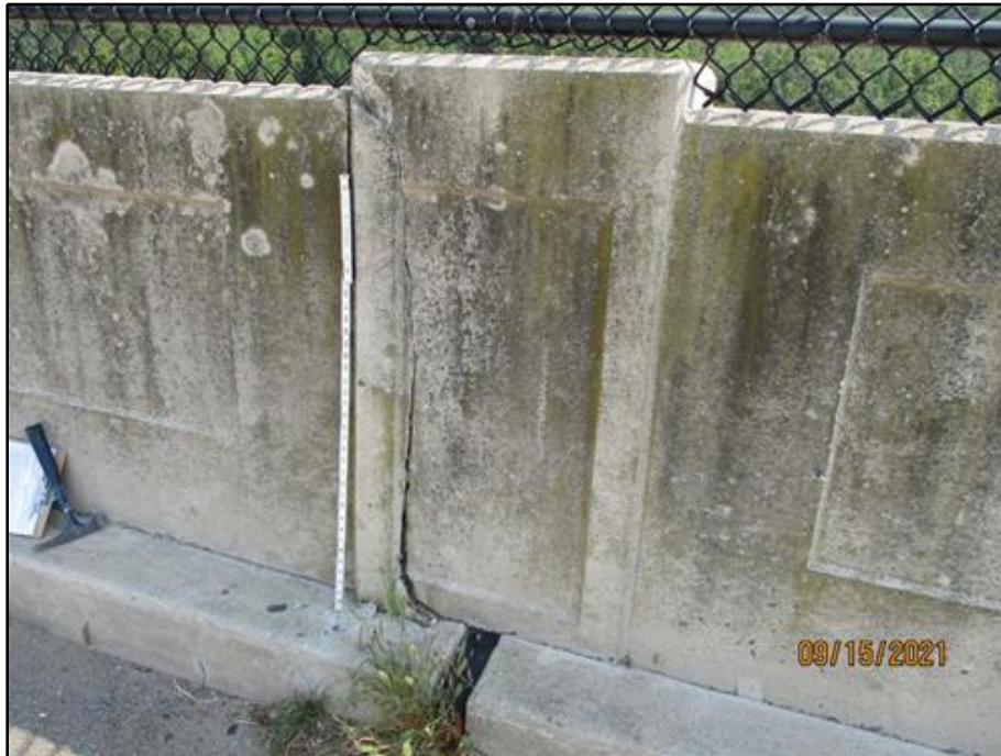
15. Cracking and imminent spall in the north face of the south parapet over Buttrass 11
