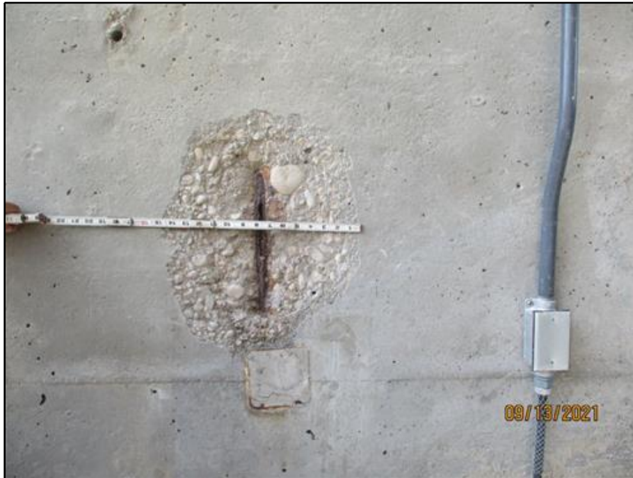
49. Typical spall around corroded electrical junction box and conduit in the buttress column (east face of Buttress 17 located 20' from the top shown)
