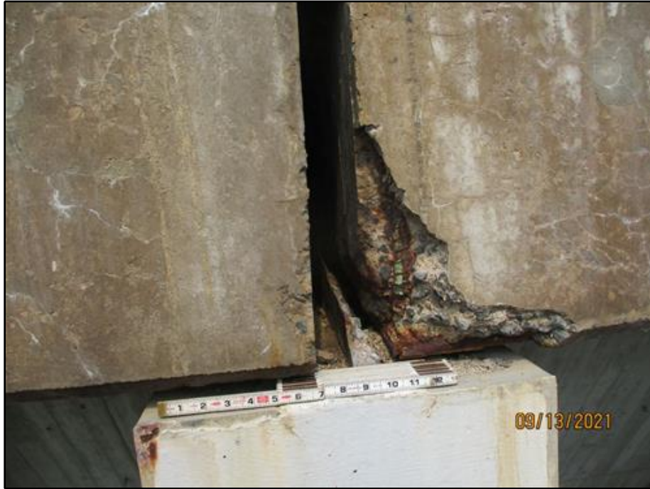
31. Full width spall on the west face of Beam 1 at the west end of Span 4 at Buttress 7
