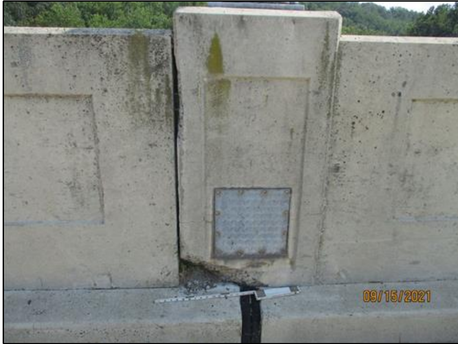
17. Spall in the north face at the base of the south parapet above Buttress 29
