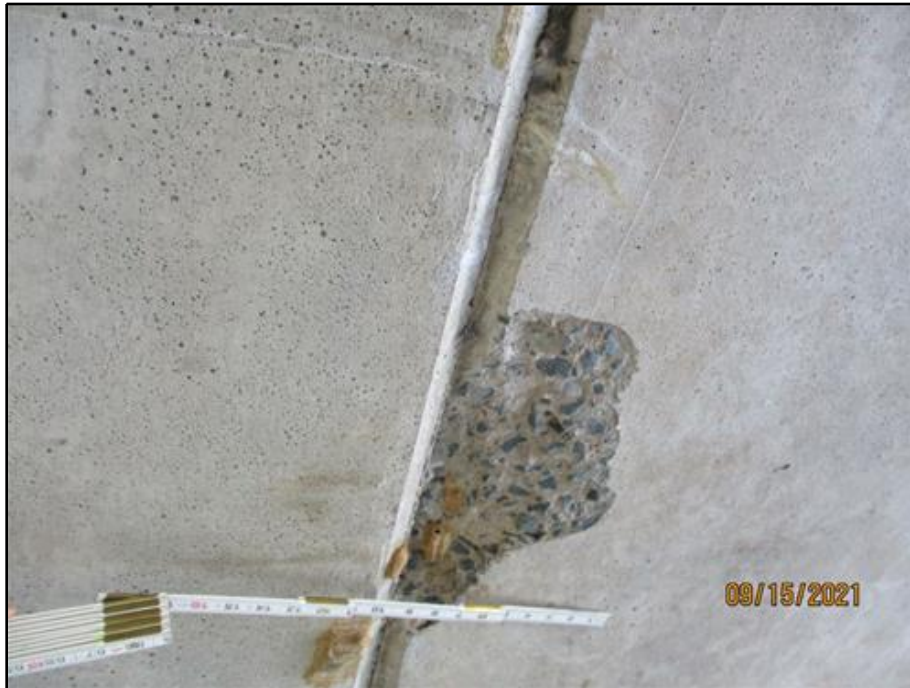
33. Spall on the bottom face of Beam 8 adjacent to Beam 9 in Span 5 near Buttress 9
