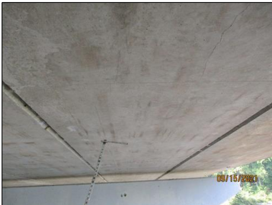
30. Two (2) longitudinal cracks in the bottom end of Beam 8 in Span 2
