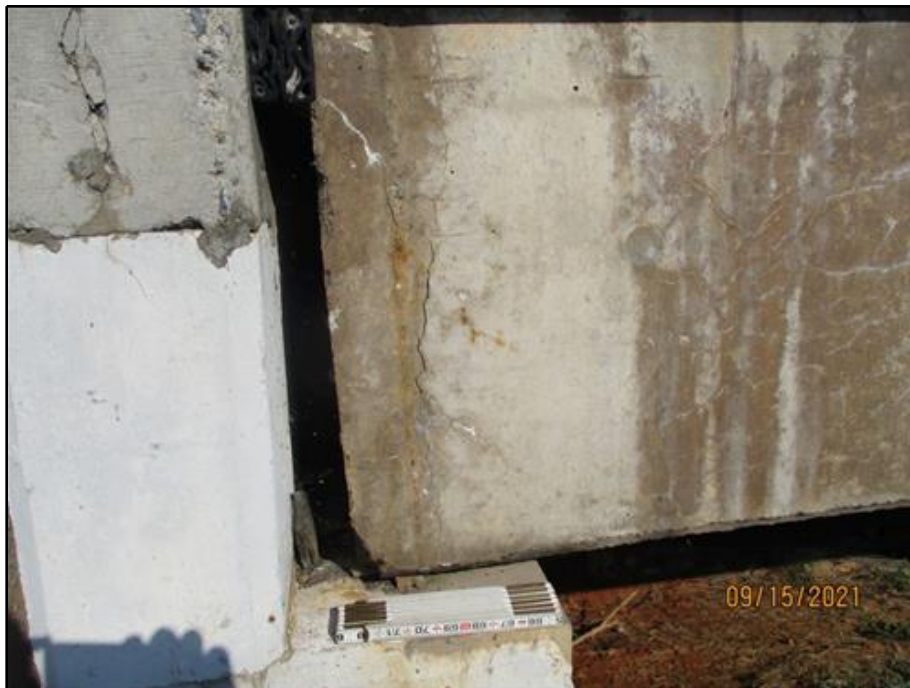
28. Vertical crack in the south face of Beam 1 at the west abutment
