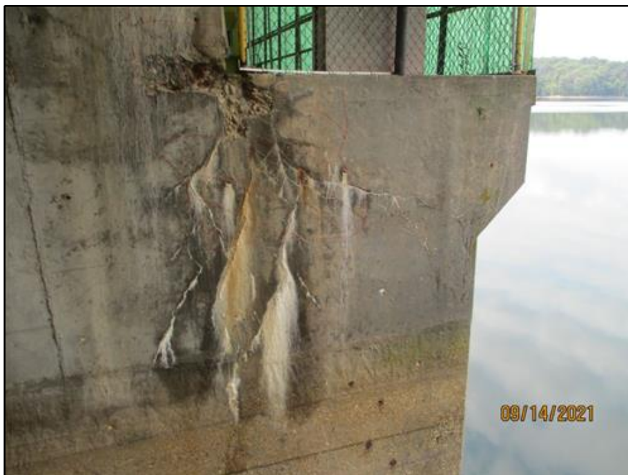
52. Spall, delaminated area, and cracks with efflorescence on the east face near the north end of Buttress 25 at the walkway support
