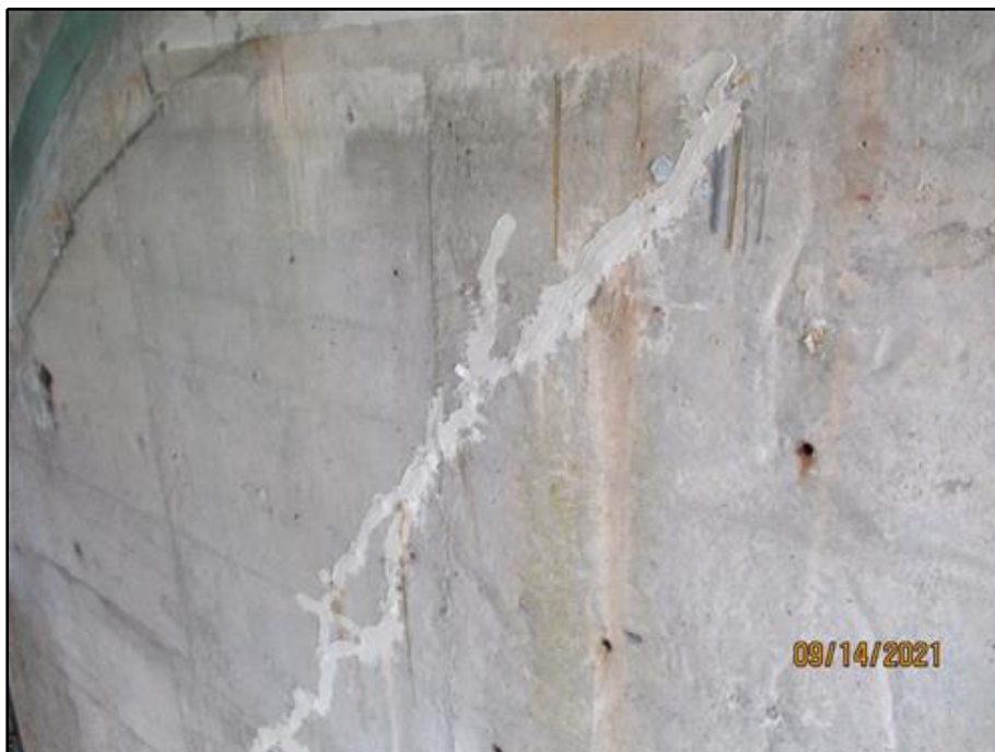
50. Typical sealed crack with strain gauge (east face of Buttress 25 shown)
