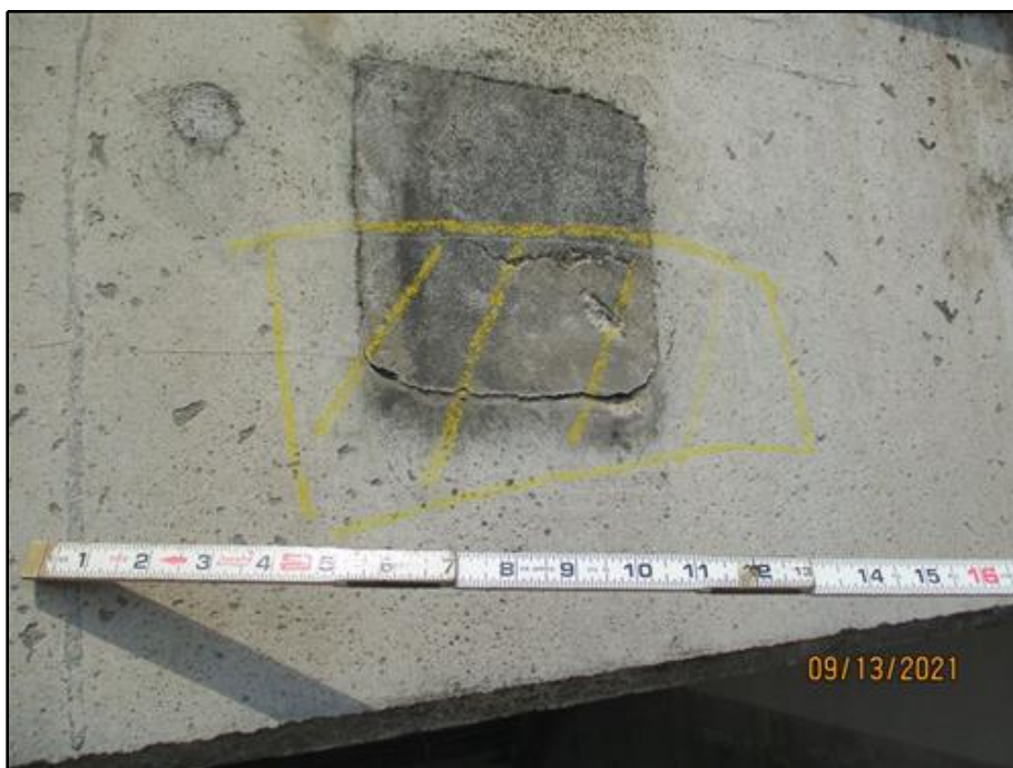
36. Delaminated tie rod grout pocket on the south face of Beam 1 at Tie Rod 3 in Span 7
