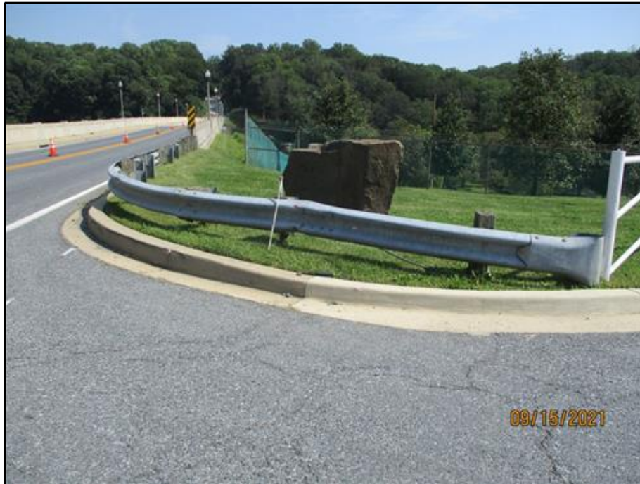
55. Impact damage at the southwest approach traffic barrier end treatment
