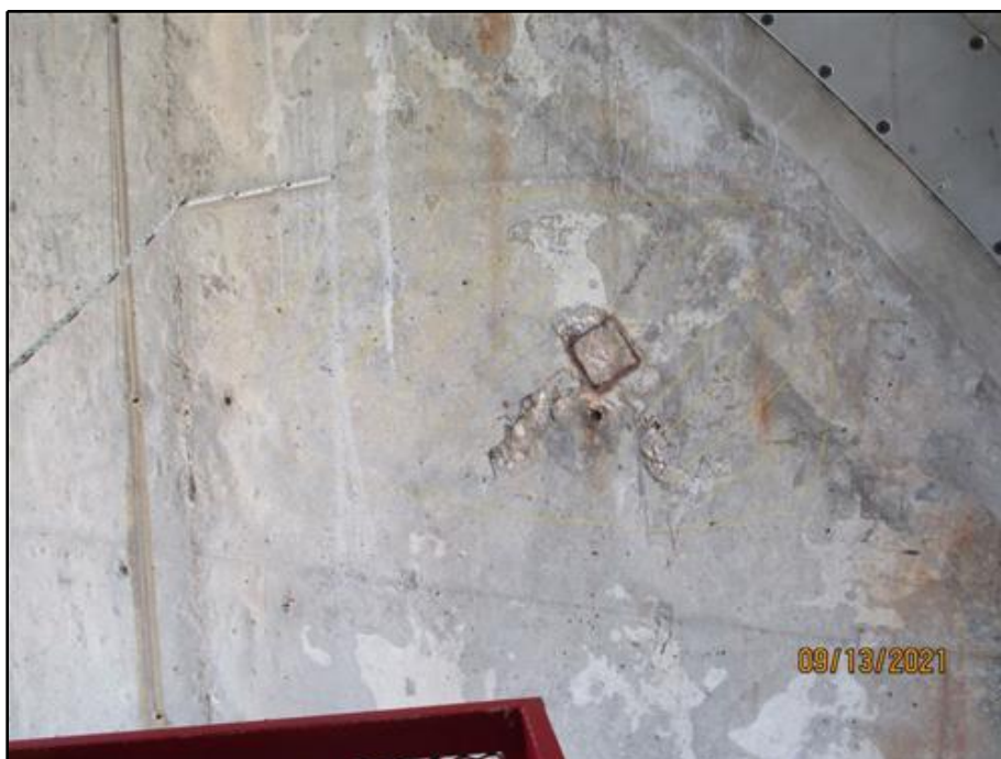
48. Delamination below the flood gate guide (east face of Buttress 15 shown)
