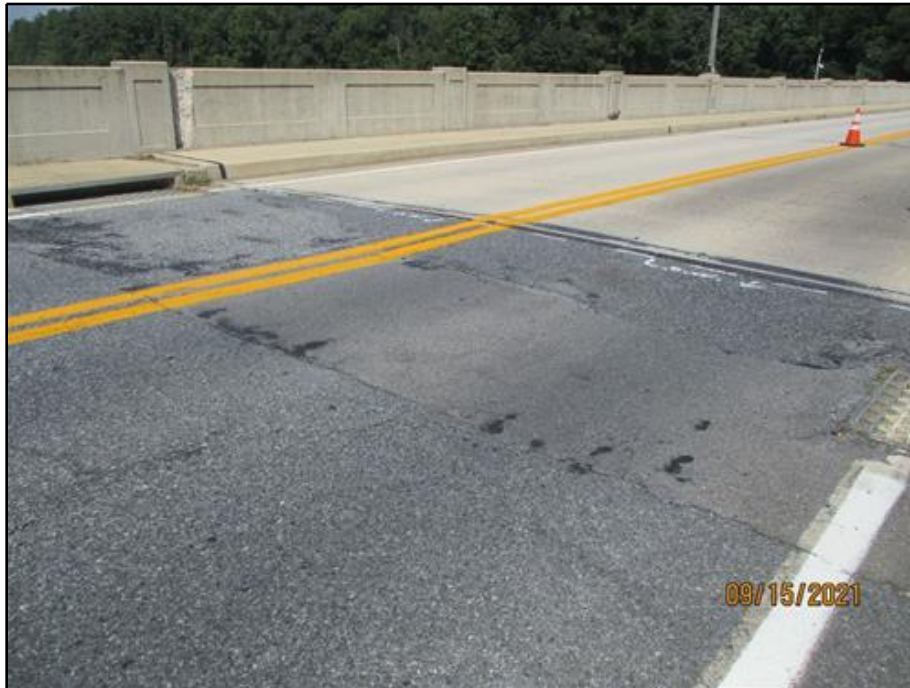
57. Full width patch at the west approach transition with settlement at the transition joint
