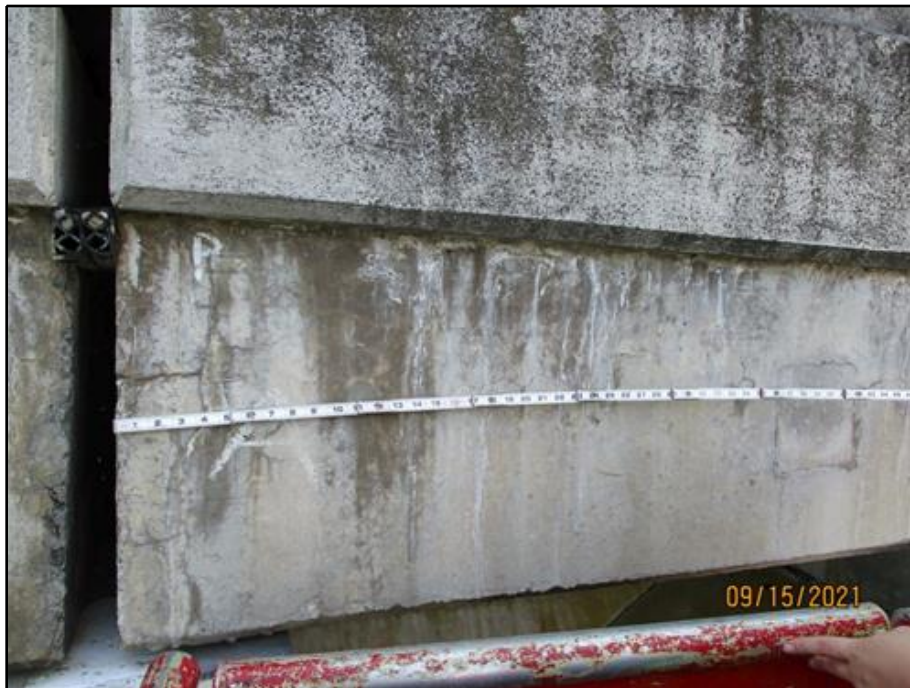
29. Horizontal crack in the north face of Beam 9 above Buttress 3 in Span 1
