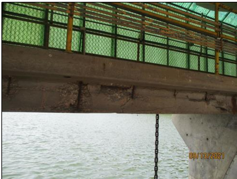
40. Typical spalling, cracks, and delamination at mid-span on the south stem of the flood gate walkway (walkway between Buttresses 19 and 20 shown)
