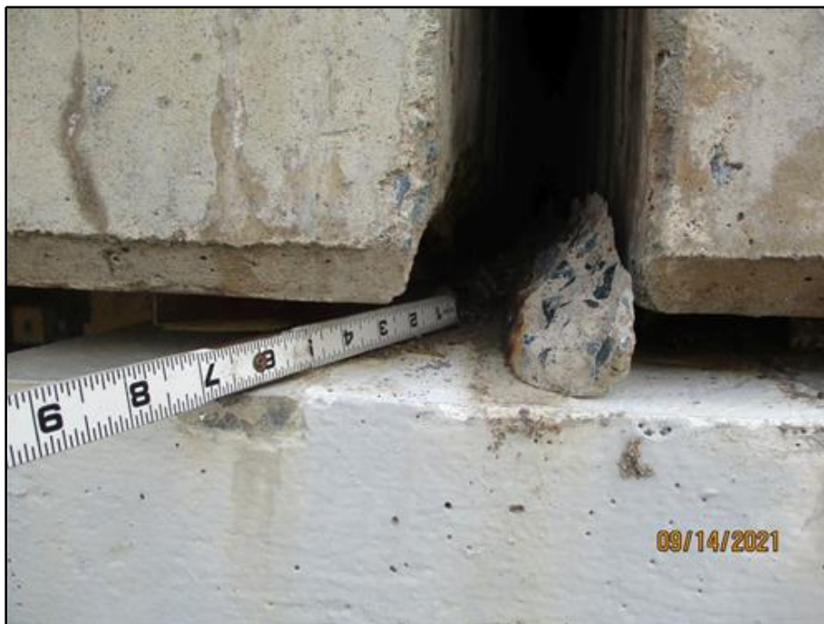
35. Corner spall on the west end of Beam 9 in Span 6 at Buttress 11
