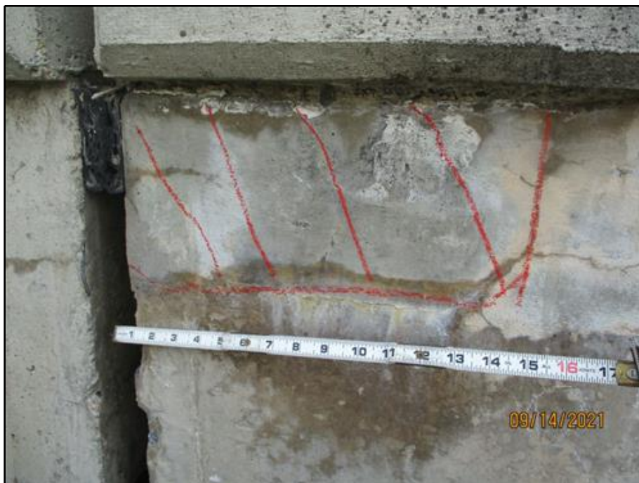
34. Delaminated patch on the north face of Beam 9 at Buttress 11 in Span 5
