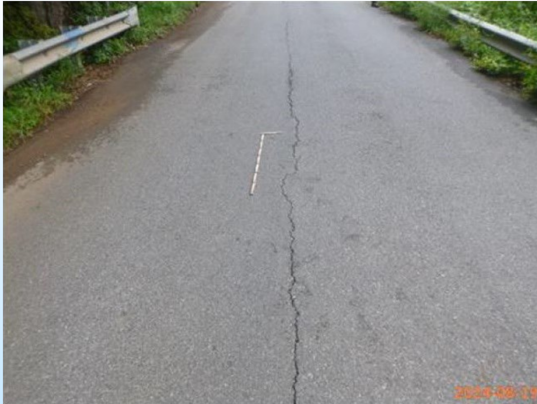
Intermittent Longitudinal Cracks along the Centerline of the Road
