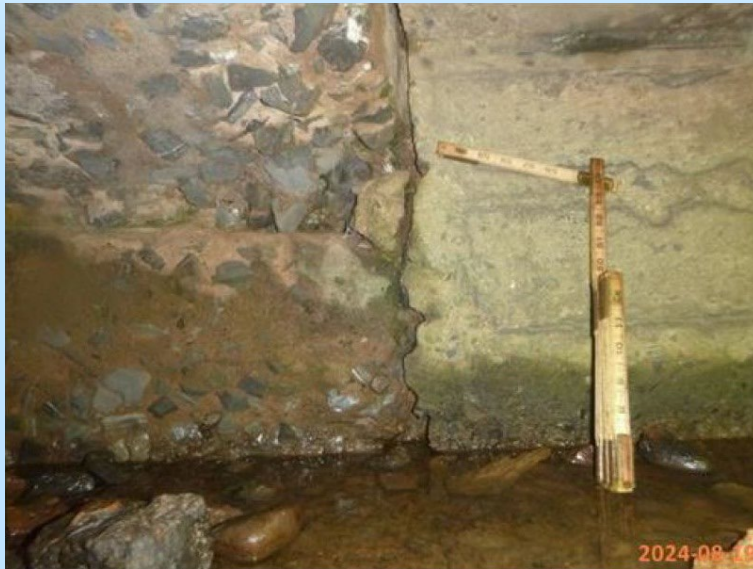
East Abutment Stem, Spalling at the Southeast Joint
