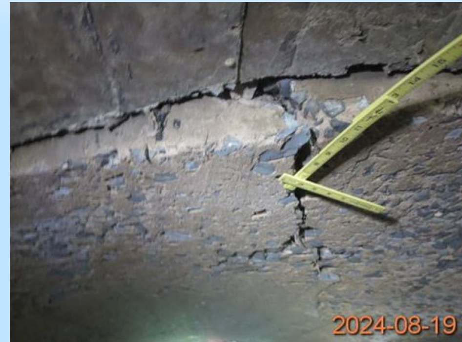
Arch Underside, North End, Diagonal Crack with Vertical Displacement at Midspan (Looking South)
