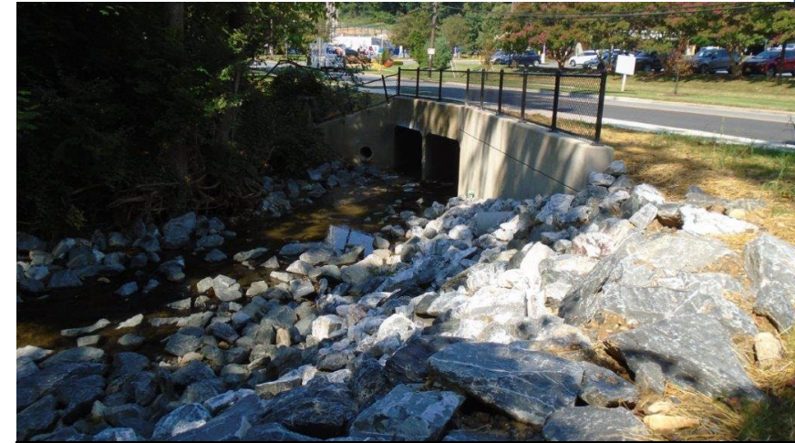
Example of Riprap Slope Protection
