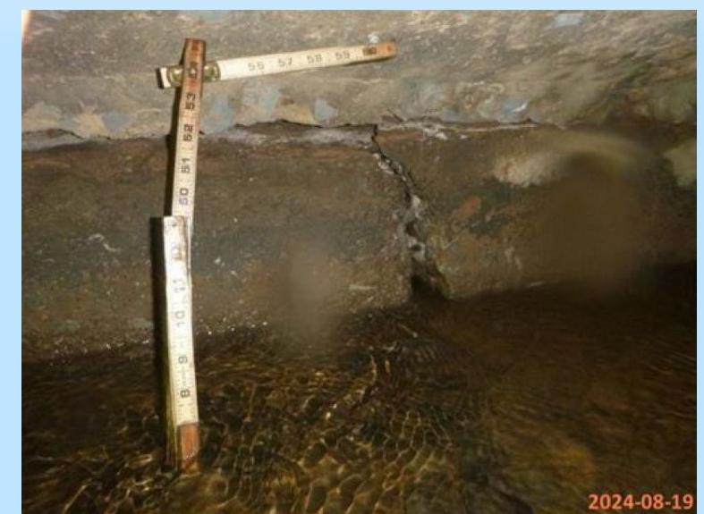
West Abutment Stem - Arch Centerline, Fracture with Vertical Displacement (Looking West)
