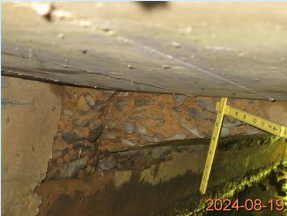
Arch Underside, North End, At the East Abutment Stem, Spalling in the Arch
