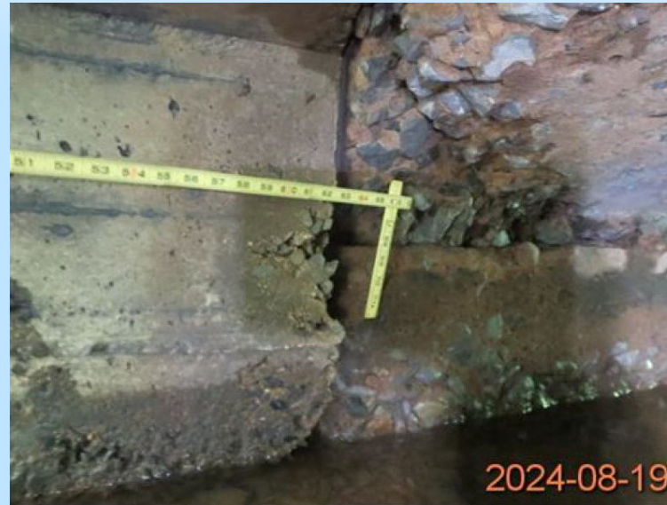
East Abutment Stem, Spalling at the Northeast Joint
