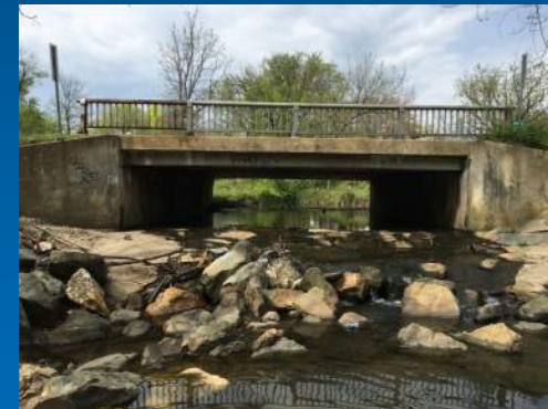
South elevation (looking upstream)
