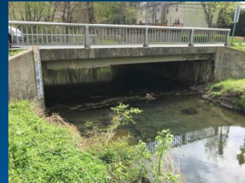
North elevation (looking downstream)
