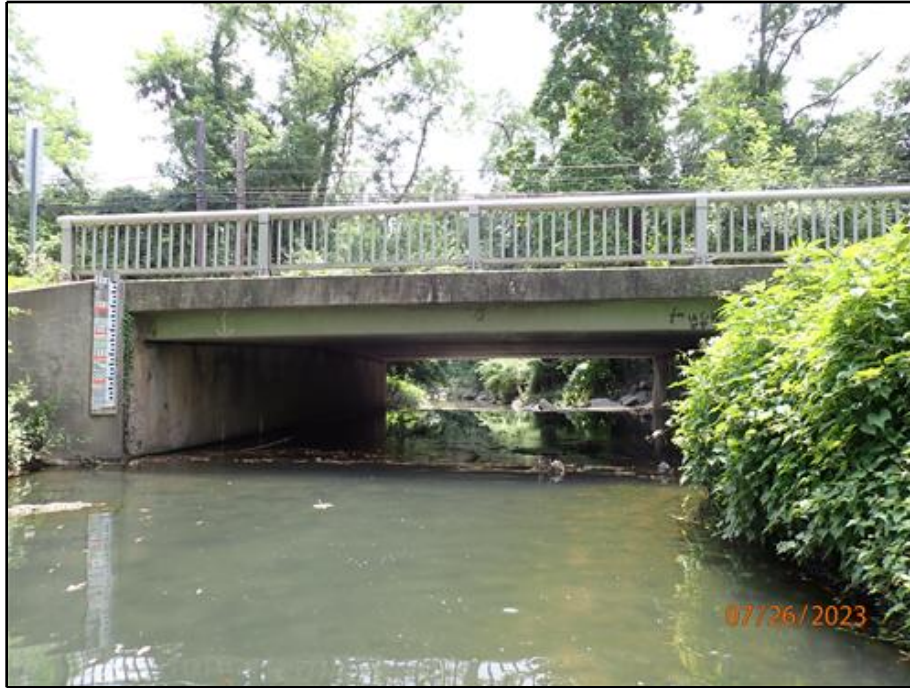
3. North Elevation (Upstream)
