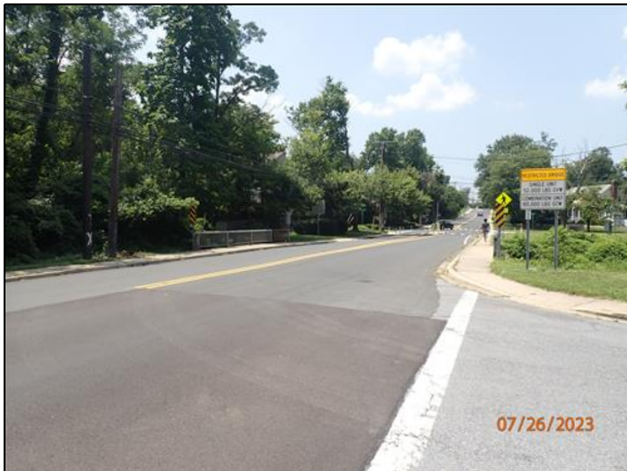
2. East Approach (Looking West)
