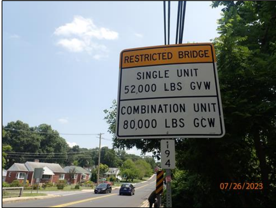
25. Load posting sign at the west approach (looking east)
