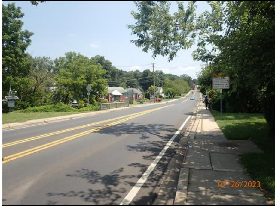
1. West Approach (Looking East)
