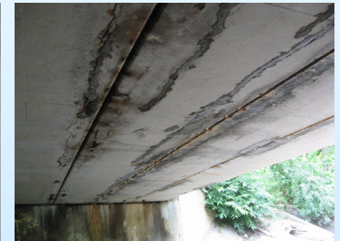
Prestressed Concrete Voided Slab Beams Spalls, Cracks and Exposed Reinforcement
