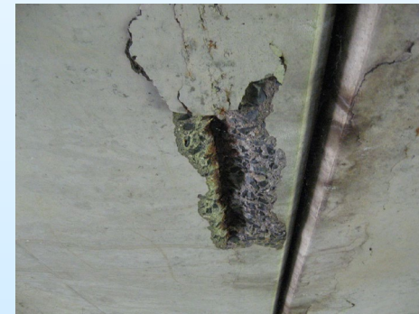
Prestressed Concrete Voided Slab Beams Spalls, Cracks and Exposed Reinforcement
