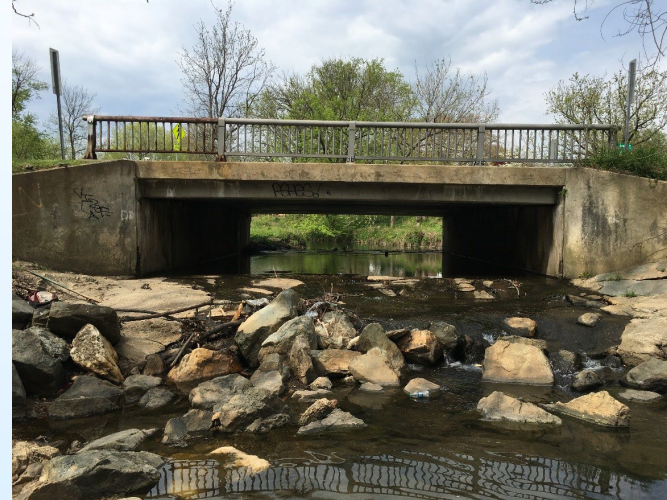
South Elevation (looking upstream)
