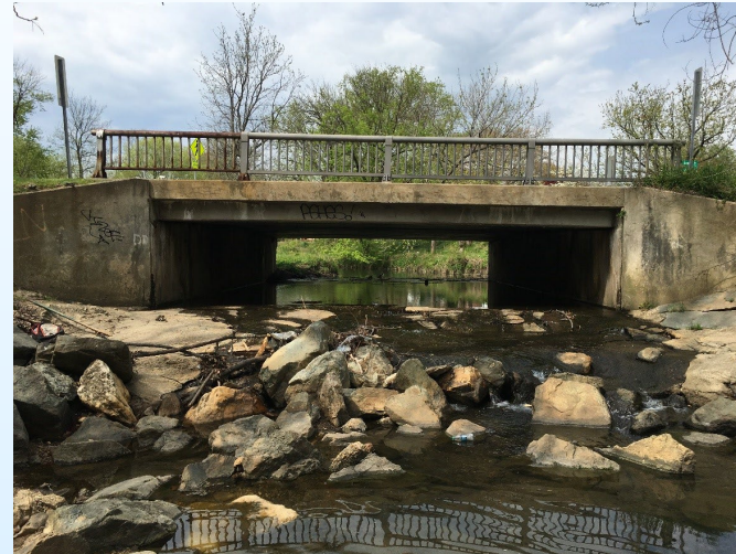
South Elevation (looking upstream)
