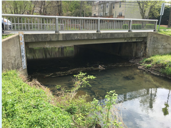
North Elevation (looking downstream)
