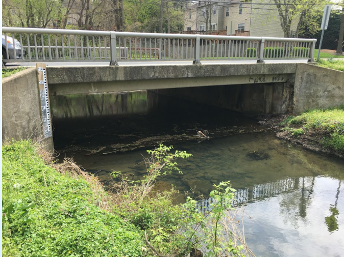
North Elevation (looking downstream)
