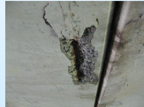
Prestressed Concrete Voids Slab Beams Spalls, Cracks and Exposed Reinforcement
