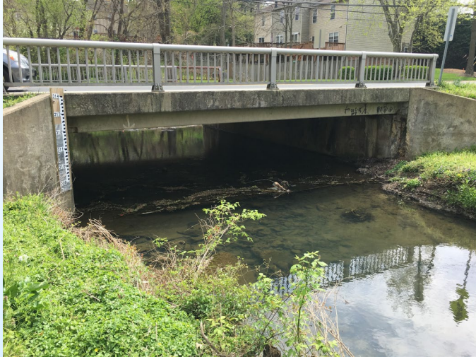
North Elevation (looking downstream)
