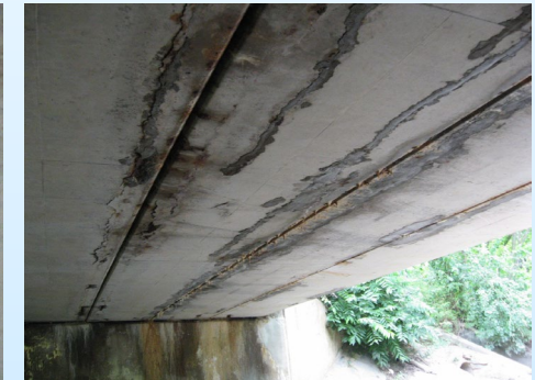
Prestressed Concrete Voids Slab Beams Spalls, Cracks and Exposed Reinforcement
