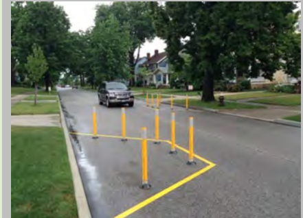
Top: speed hump. Second from top: bump-out Third from top: mini roundabout Bottom: chicane
