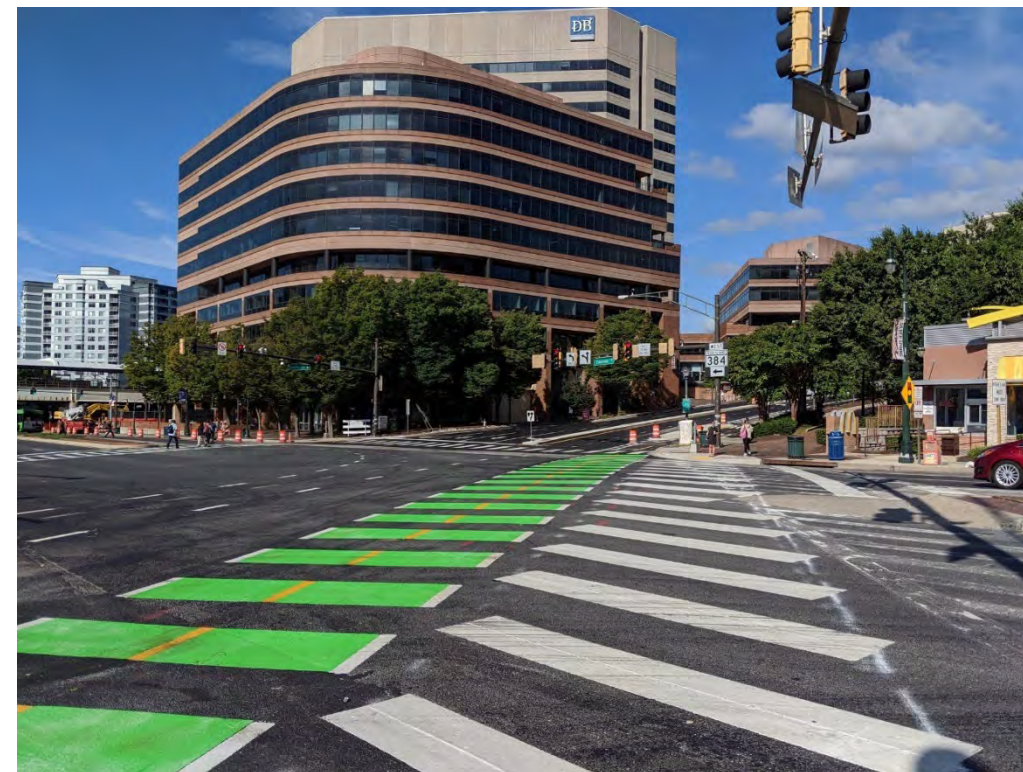
Figure 27 - Green paint conflict zone at Second Ave / Wayne Ave and Colesville Road (MD 384)
