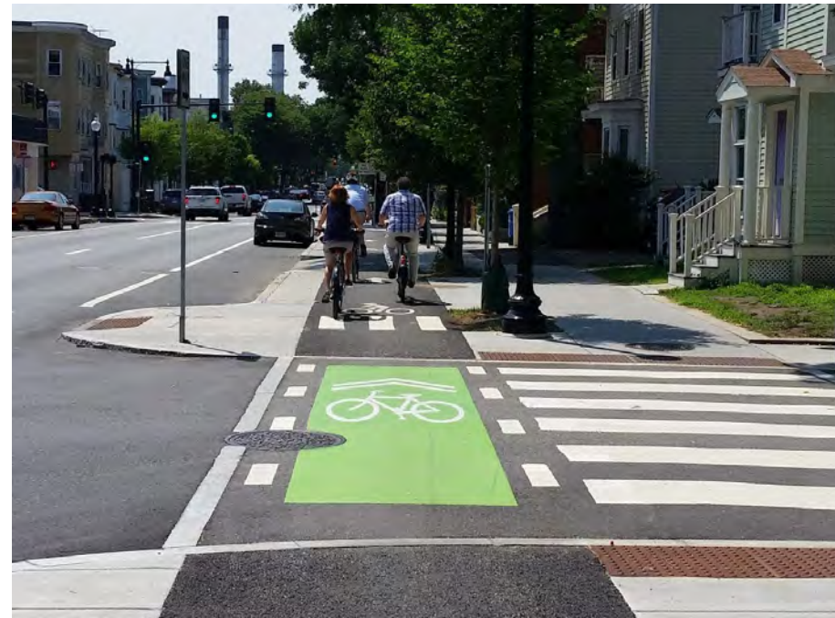
Figure 29 - Example treatment at side street intersection with a one-way cycle track in Cambridge, MA.
