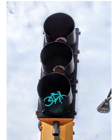
Figure 24 - Bicycle signal at Second Ave / Wayne Ave & Colesville Road (MD 384)
