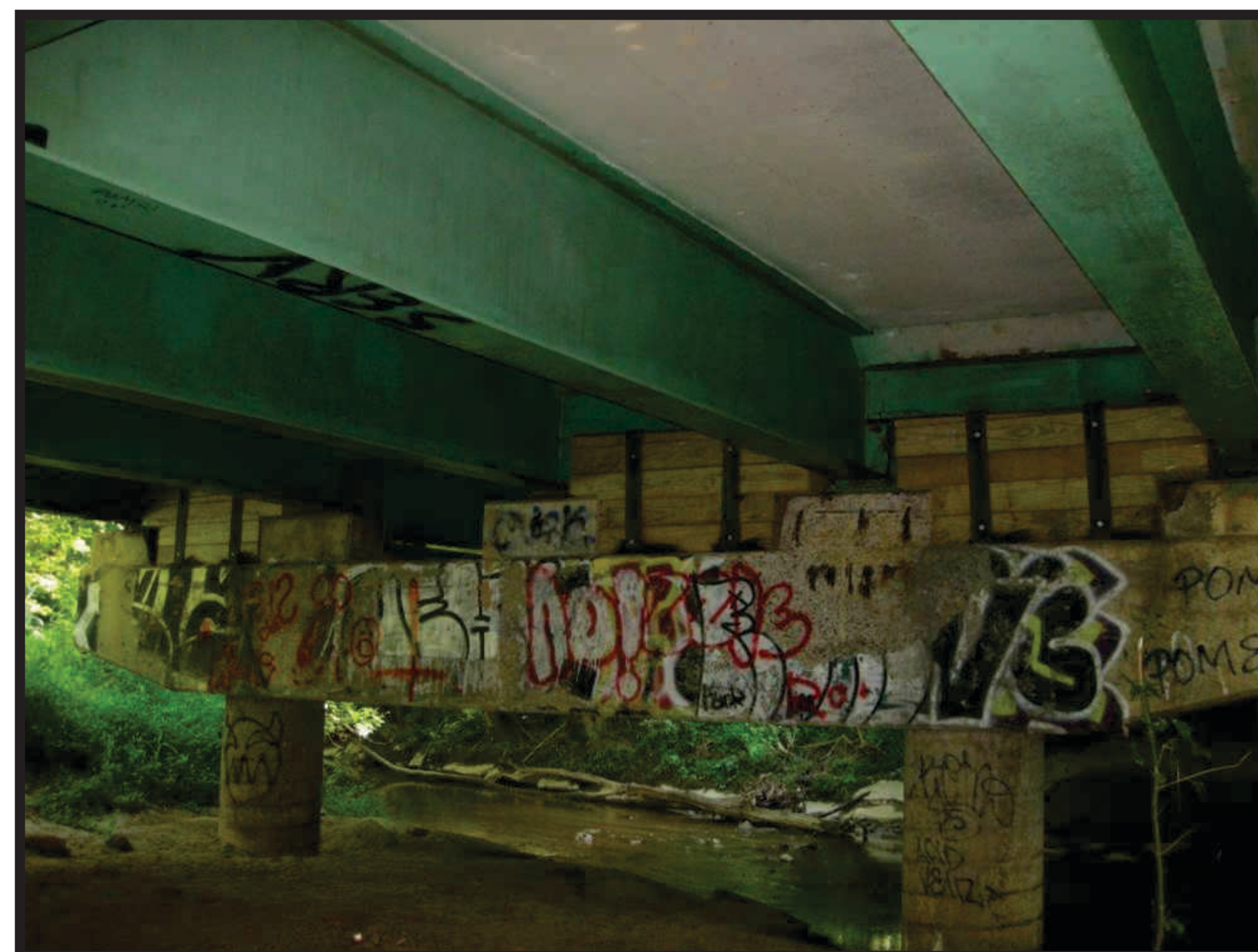
Timber blocking repairs
