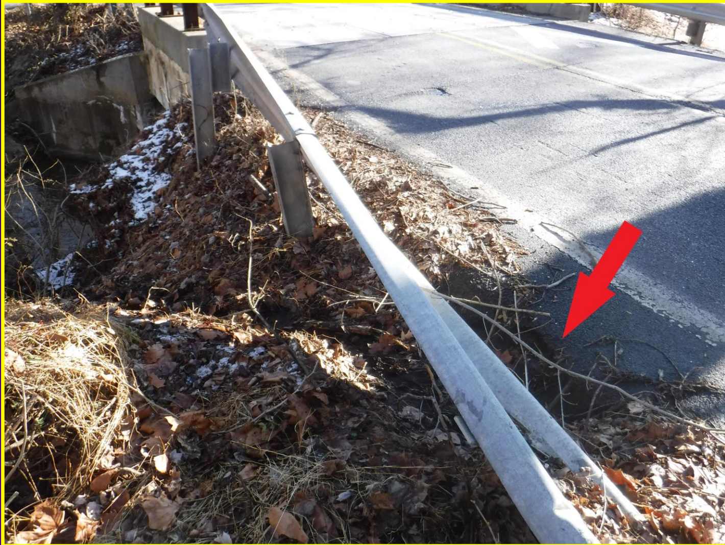
Erosion Along the Shoulder at the Northwest Embankment
