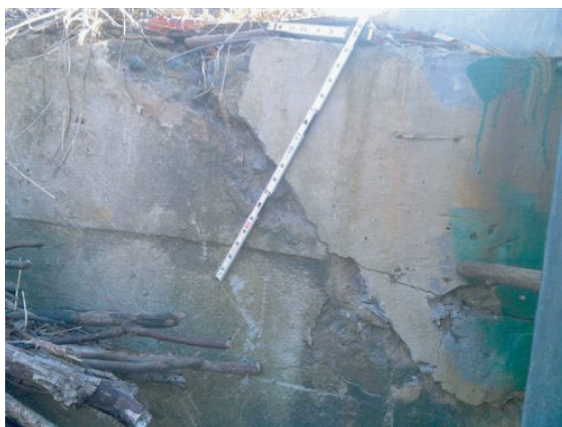
Cracks and Spalls in Concrete Wing Walls
