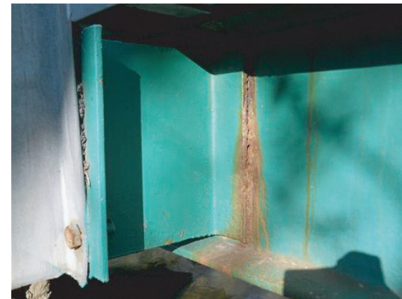
Cracked Railing Post Bracket Welds
