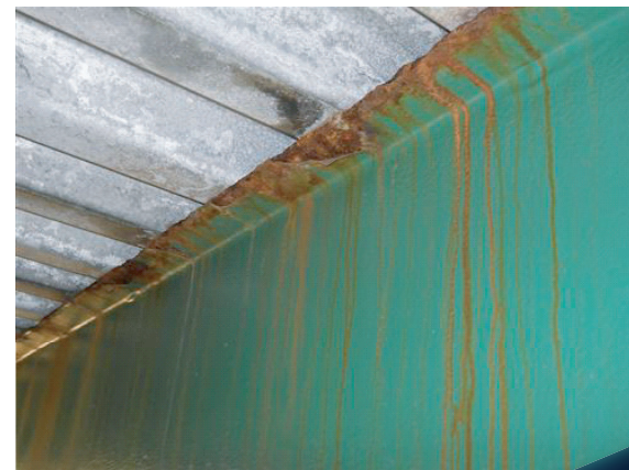
Rusting Along Beam Flanges
