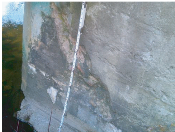
Cracks and Spalls in Concrete Wing Walls
