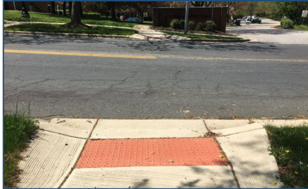
(a) ADA Ramp south of Bantry Way (north)
