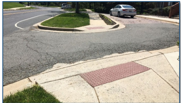
(b) Ramp at Towne Center Place Driveway
