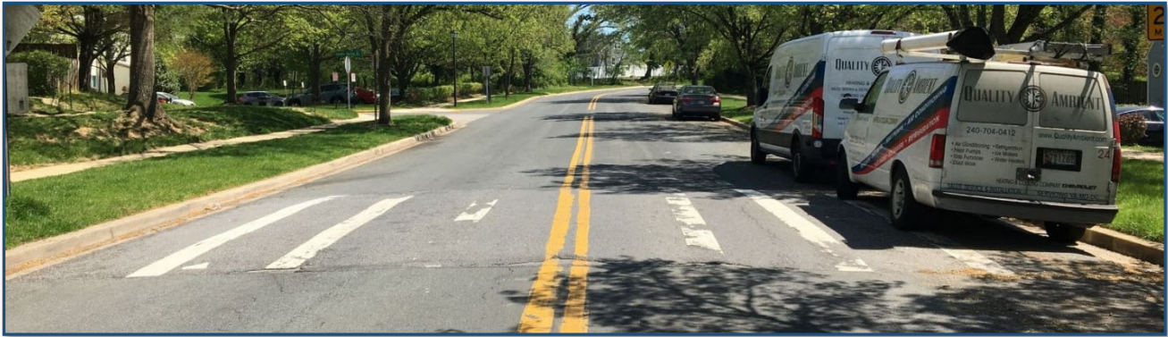
(a) Looking east
