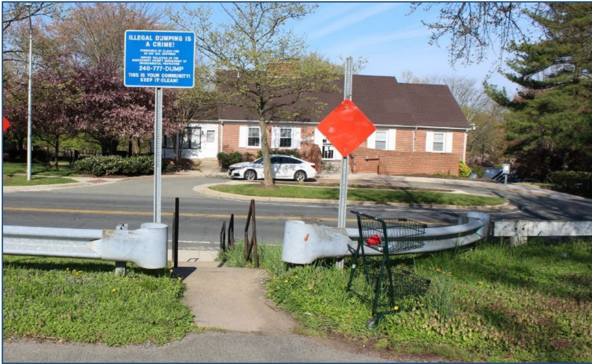
Figure 2-2: Community Maintenance Building from N. High Street
