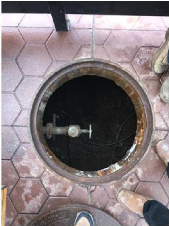
Figure 4-7 | Site Visit Photo – Platform Manhole Removed with Standpipe Visible
