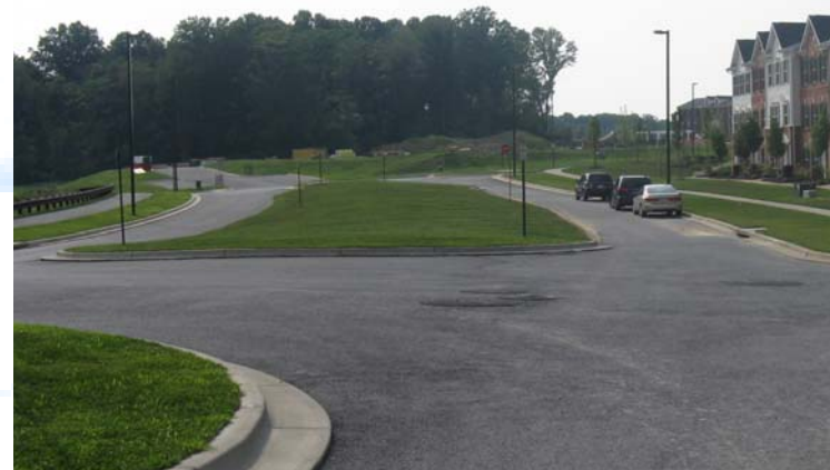
Existing Roberts Tavern Drive between Latrobe Lane and Observation Drive.
