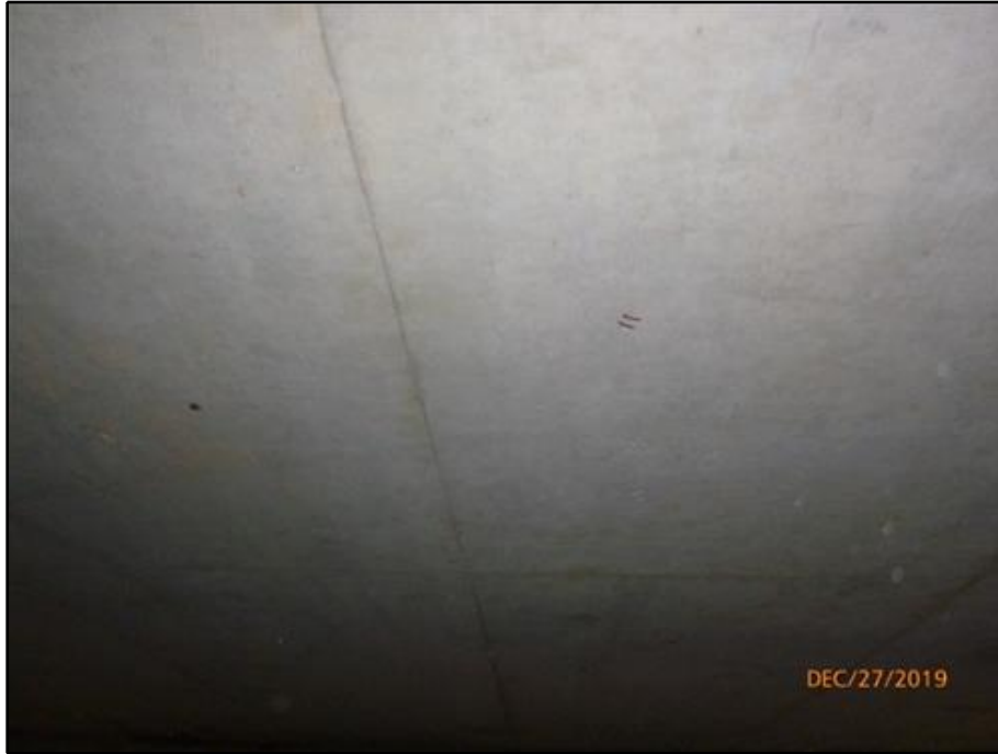
9. Typical underside of superstructure
