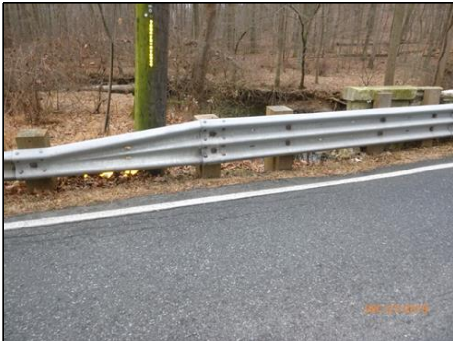
30. Typical three beam transition (northeast shown)
