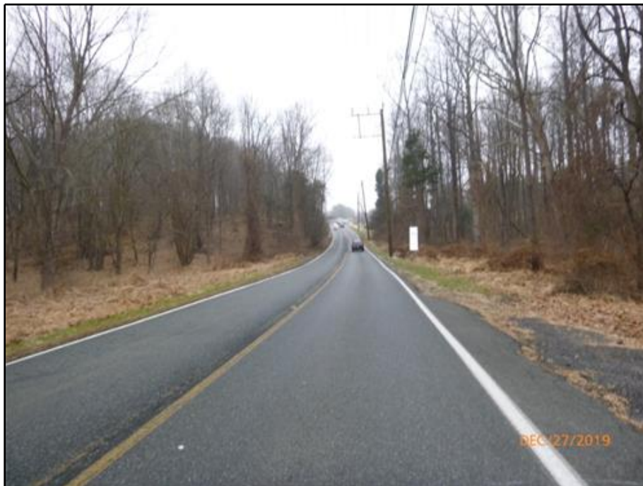
2. North Approach Looking North
