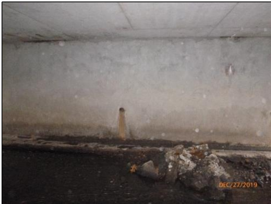
10. North Abutment Elevation
