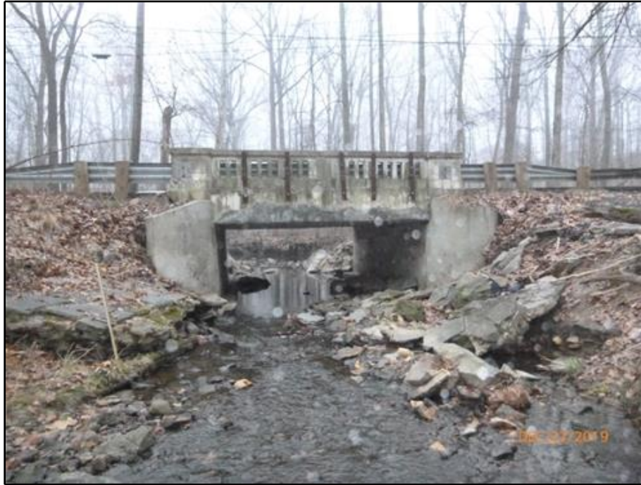
7. West (Upstream) Elevation
