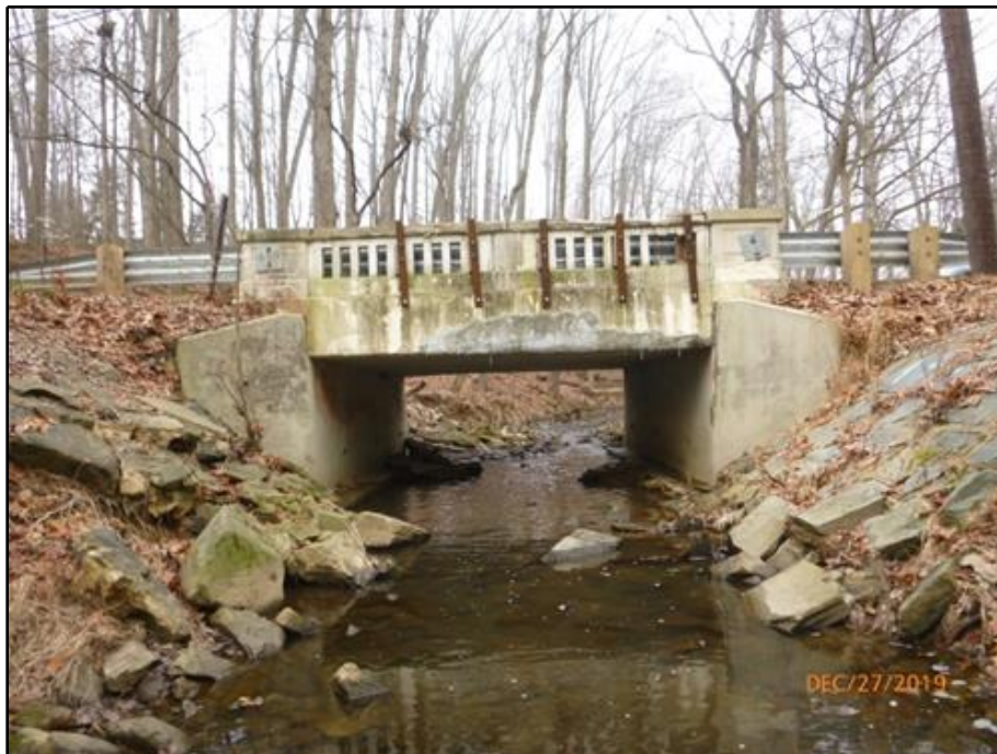
8. East (Downstream) Elevation
