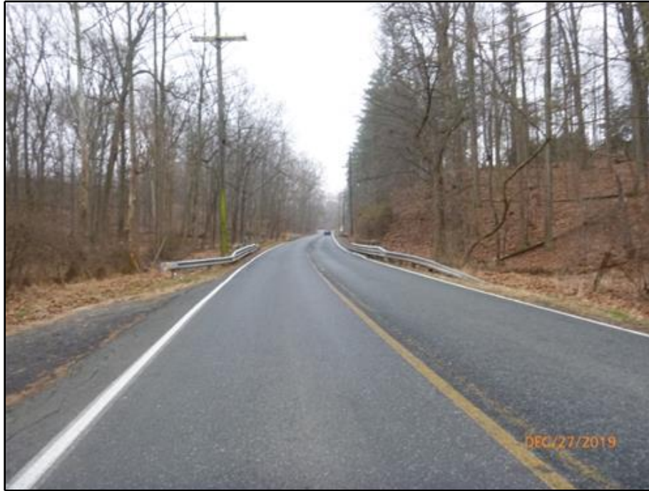
1. North Approach Looking South
