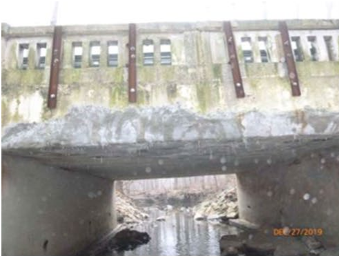
Delaminated Concrete
