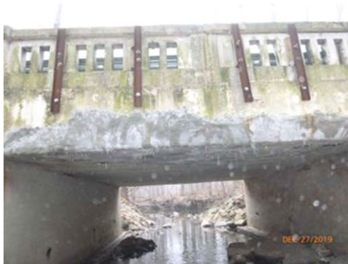
Delaminated Concrete
