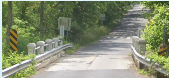
Topside Superstructure (looking east)
