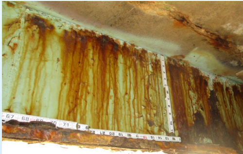
Peeling Paint, Rust Staining and Heavy Corrosion at Beams
