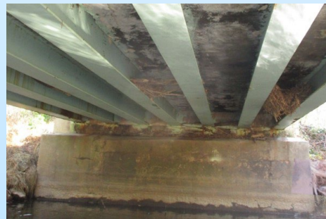
East Abutment and Underside Superstructure
