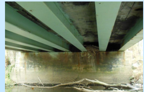
West Abutment and Underside Superstructure
