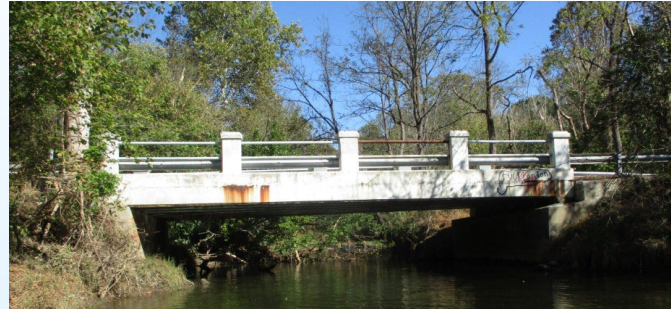
South Elevation (downstream)
