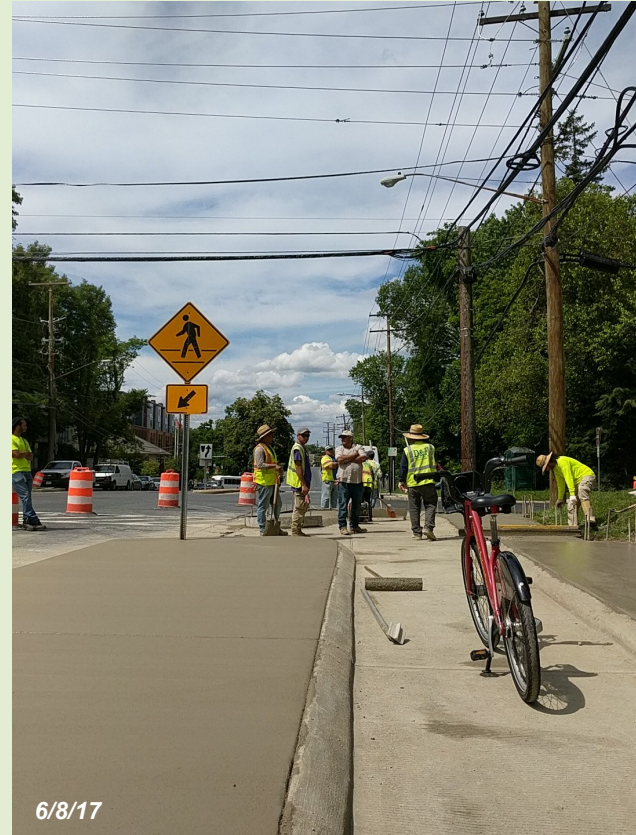
The bikeway will go behind these corner islands at Spring Street and First Avenue, slowing turning vehicles and shortening pedestrian crossing distances.
