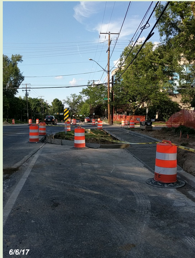
The bikeway will go behind these corner islands at Spring Street and First Avenue, slowing turning vehicles and shortening pedestrian crossing distances.
