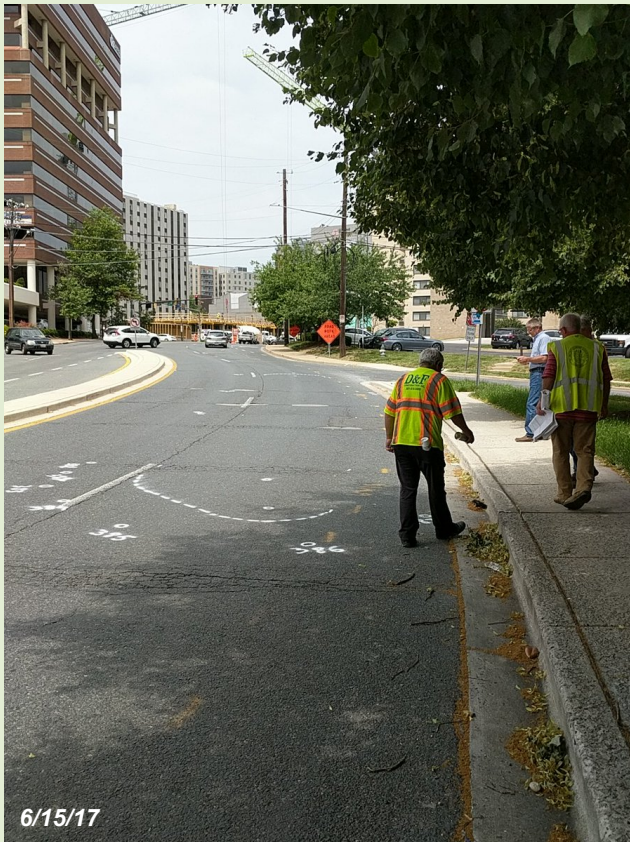
Workers are marking the location of a floating bus stop along Spring Street at Ellsworth Drive. Here, the bikeway will go between the bus platform and the sidewalk, meaning the bus won't need to block the bike lane while at the stop.
