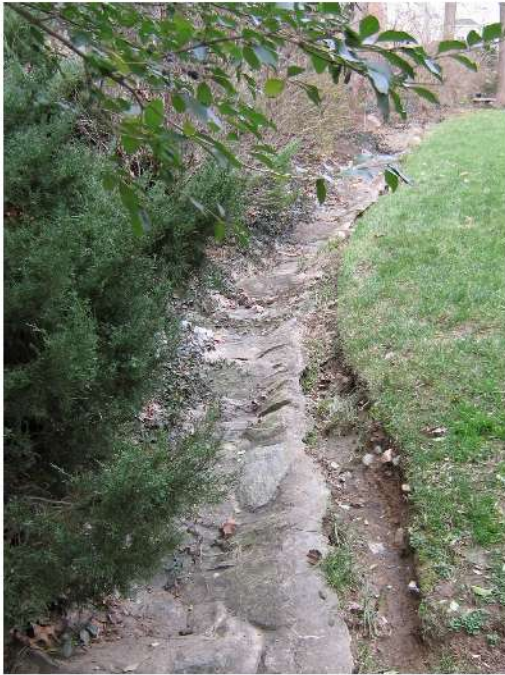
Photo 2 – Concrete and Stone Ditch at 5400 Tuscarawas Road
