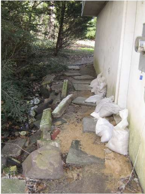
Photo 1 – Drainage Ditch at 5409 Wehawken Road
