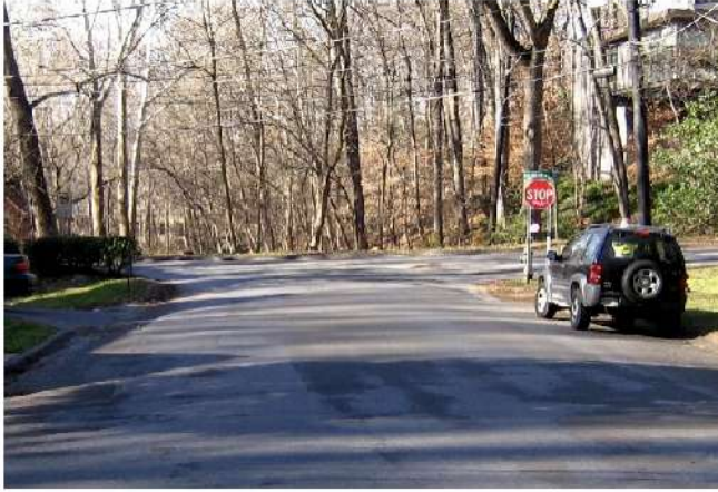
Photo 16 – Intersection of Walhonding and Tuscarawas
