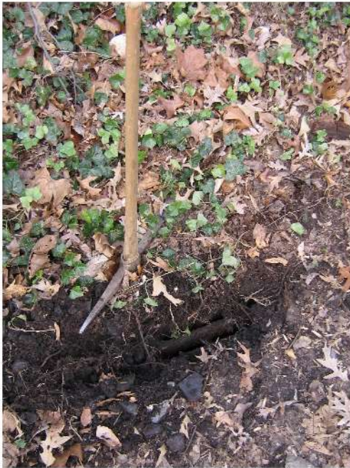
Photo 4- Covered Inlet along Walhonding Road
