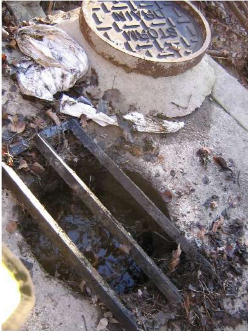
Photo 12 – Manhole Located Behind 5104 River Hill Road
