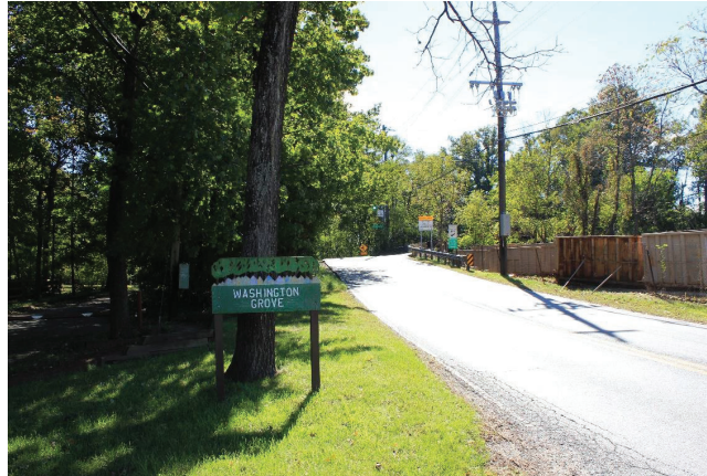
View 5A: Looking southeast along Railroad Street from its intersection with Brown Street. The Railroad Street corridor encompasses the Humpback Bridge and its approaches (center of image).
