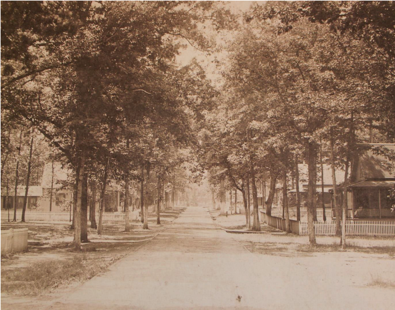
Figure 7: Early view of Grove Avenue, no date. [Washington Grove Archives]
