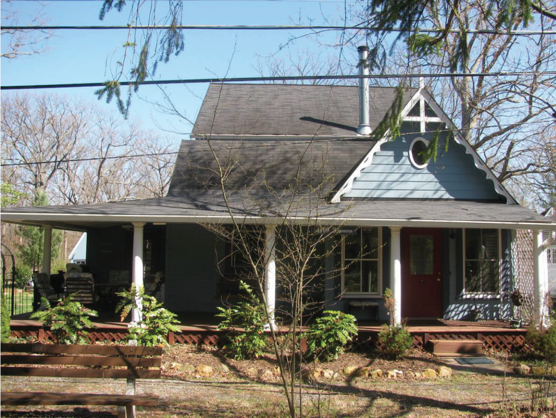
MD_MontgomeryCounty_WashingtonGroveHD_0026.tif 409 Fifth Avenue, looking southeast
