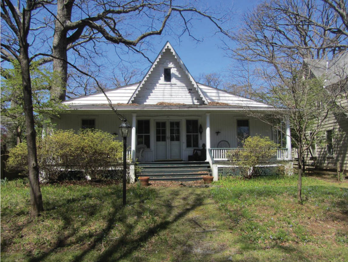
MD_MontgomeryCounty_WashingtonGroveHD_0023.tif 112 Grove Avenue, looking northwest
