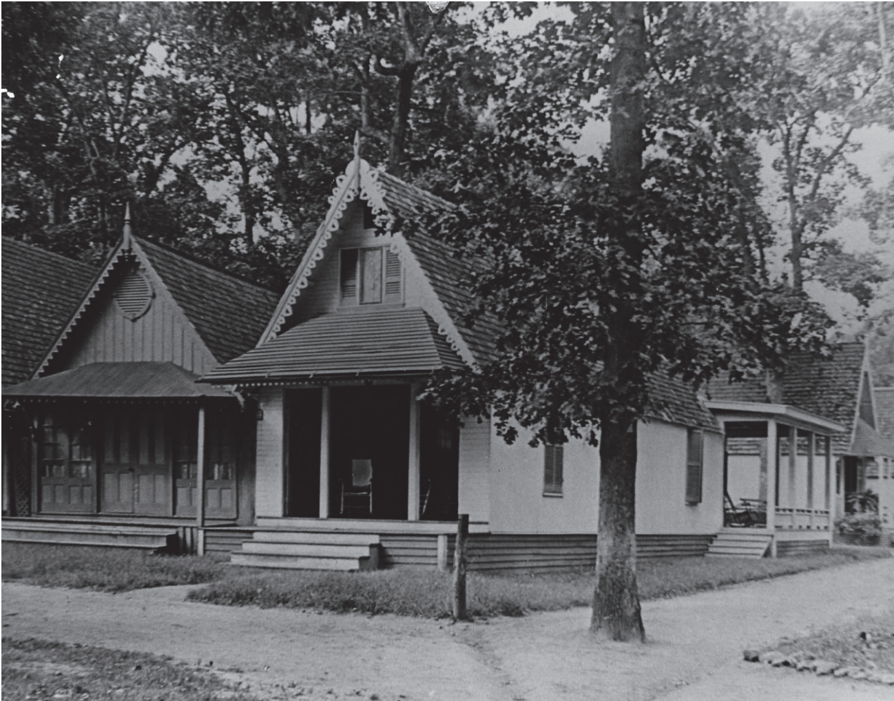
Figure 8: Undated view of Washington Grove showing two forms of early cottage construction and design. [Washington Grove Archives]
