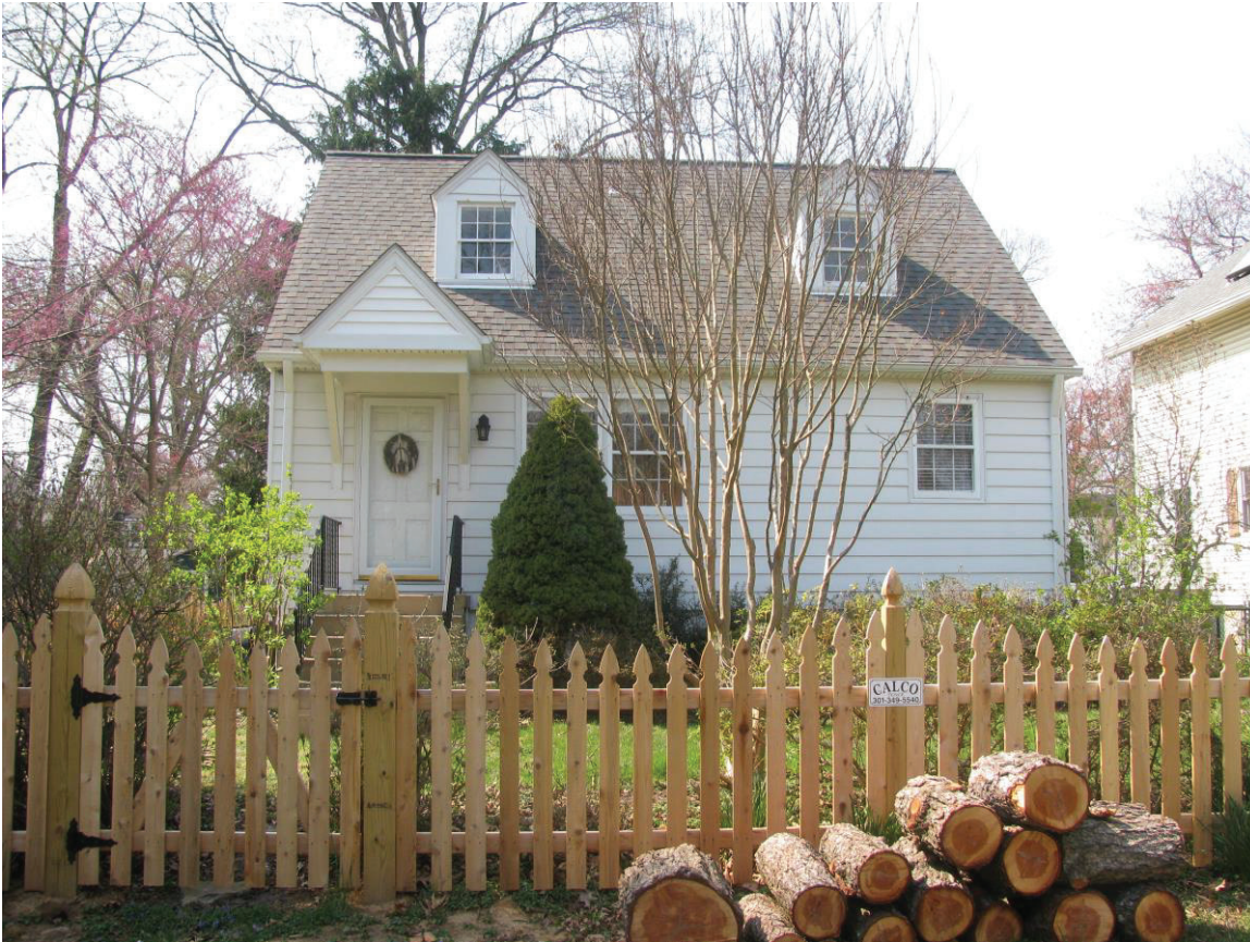
MD_MontgomeryCounty_WashingtonGroveHD_0035.tif 106 Pine Avenue, looking northwest
