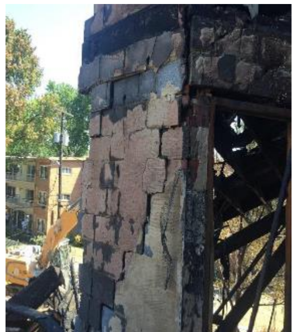
Interior load bearing URM Wall 8701 – unstable
