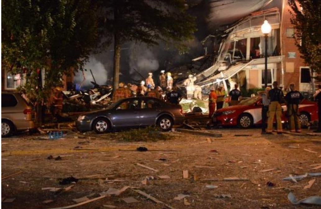
Side Alpha of 8701 Arliss Street. A small part of the debris field is in the foreground. The collapsed area is where the original entryway and stairwell to the building were.
