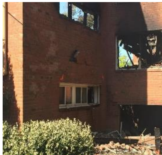
Side Charlie Wall – Cracks and outward bowing
