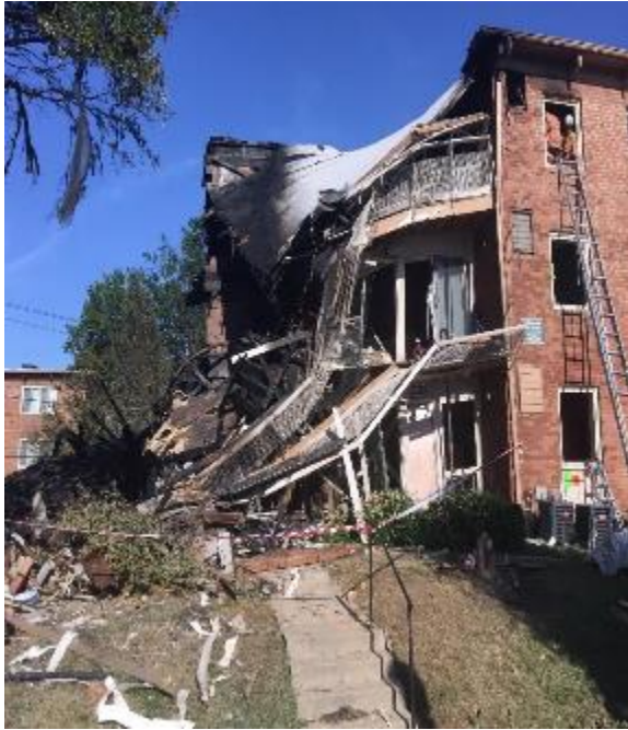
"Lean To" collapse – Side Alpha 8701 – unstable roof Compromised
