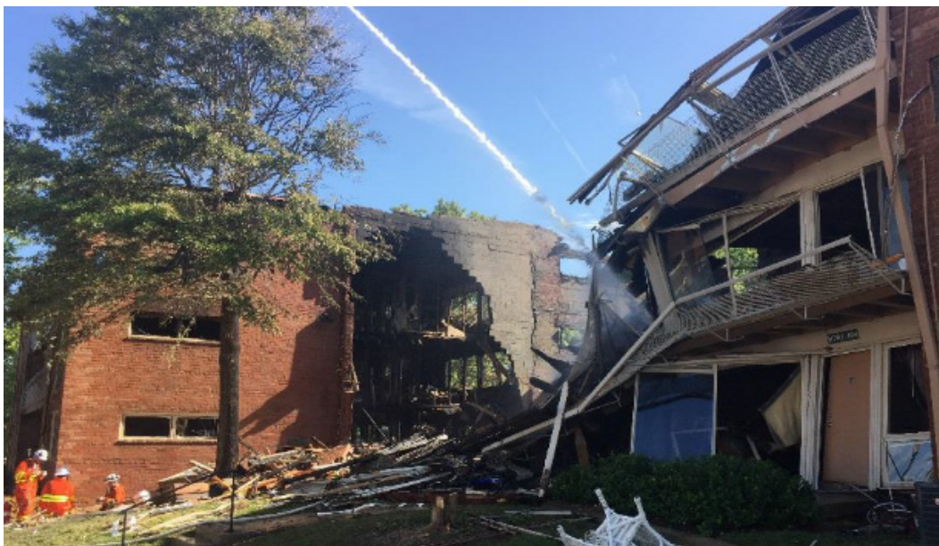
The fire wall that was blown out between 8701 on the right, and 8703 on the left.
