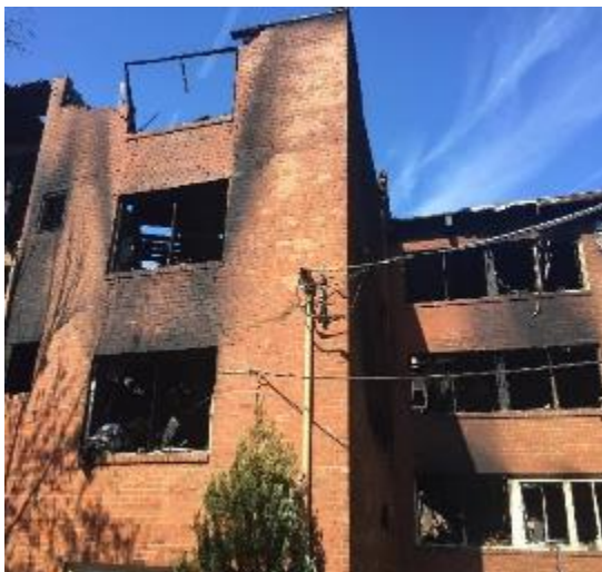
Side Charlie Wall – Cracks and outward bowing noted noted
