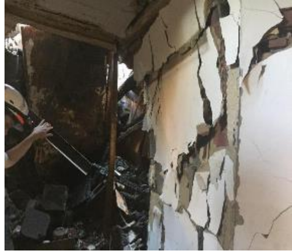
Failing Interior URM Wall – Stairwell - 8701
