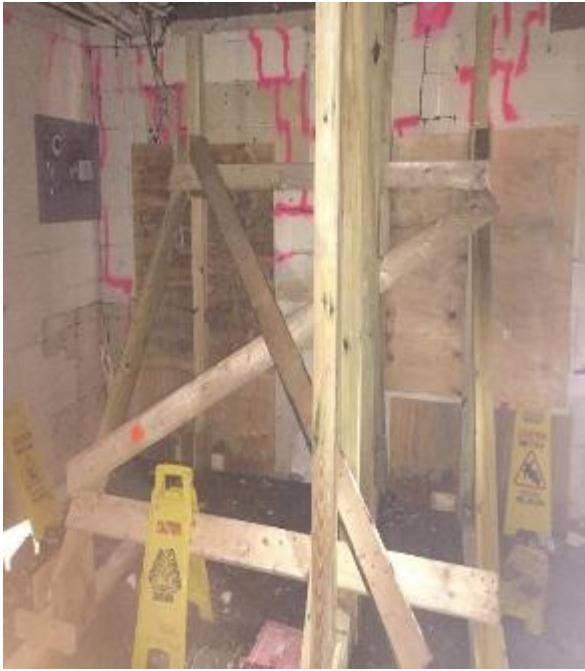
Vertical Shore / Raker Shore interior wall – 8701 Terrace
