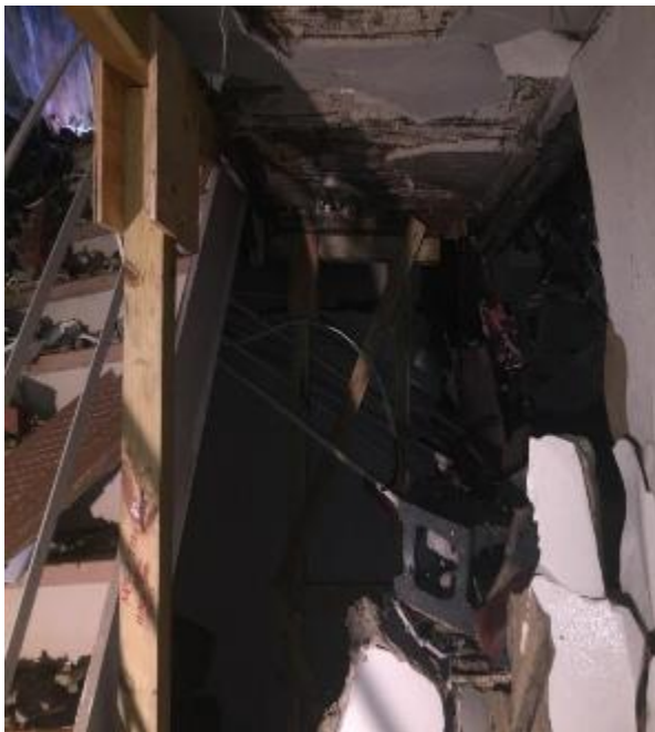
T Shore & 2 Post Vertical – Stairwell 8701 - Terrace Terrace
