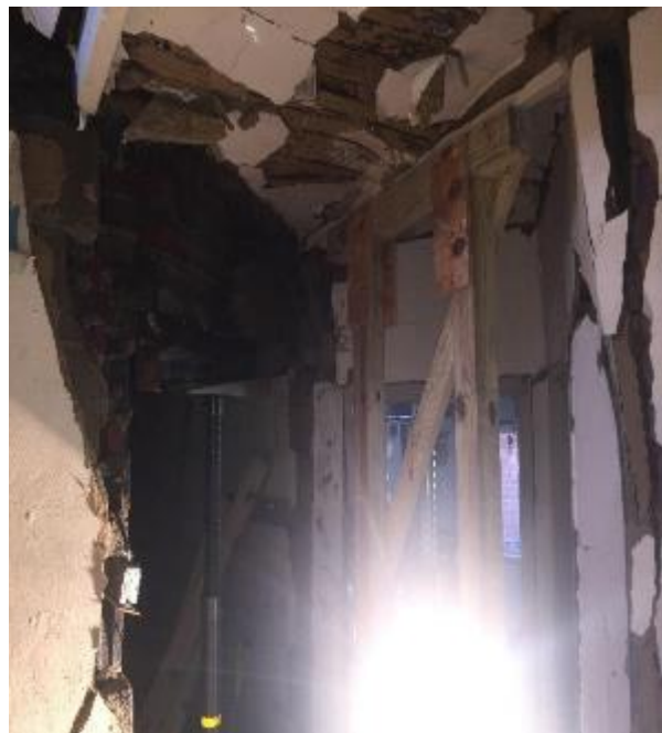
Strut to protect doorway / 2 post vertical – 8701 -
