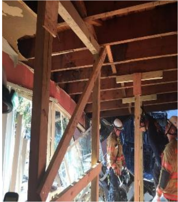
2-Post Vertical & T Shore – Second Floor - 8701
