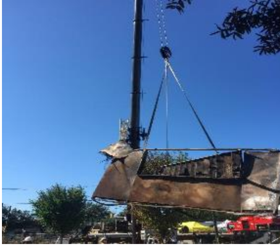
Removal of Stairwell Structure
