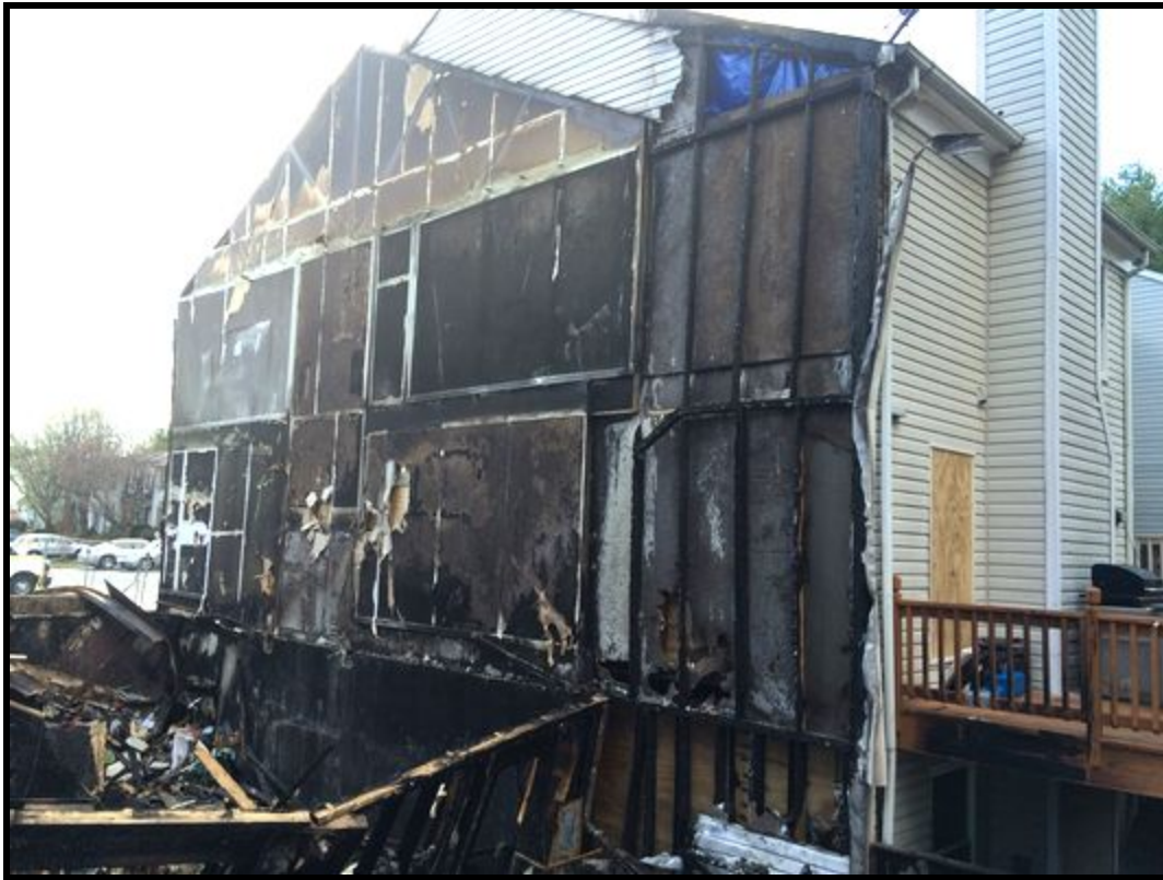
A view of the aftermath from Side Charlie note the basement level exterior wall leaning outwards.
