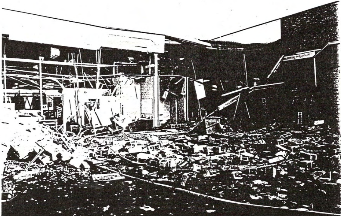
AREA TO RIGHT OF CENTER IS REAR OF GRAPE & GRAIN - 190223 WATKINS MILL ROAD - GAS LEAK & FIRE IN CORNER TO REAR OF THAT STORE - NOTE HANDLINE UNDER DEBRIS.
