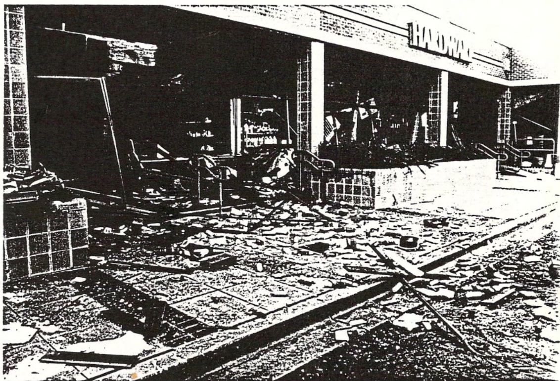
OVERVIEW OF SIDE ONE OF STORES AFFECTED BY EXPLOSION. NOTE AMOUNT OF DEBRIS THAT FORCEFULLY BLEW OUT FRONT OF STORES.
