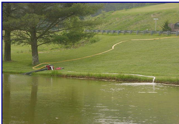
One fill site with 2 fill stations. One Engine company and a portable pump 100ft apart.
