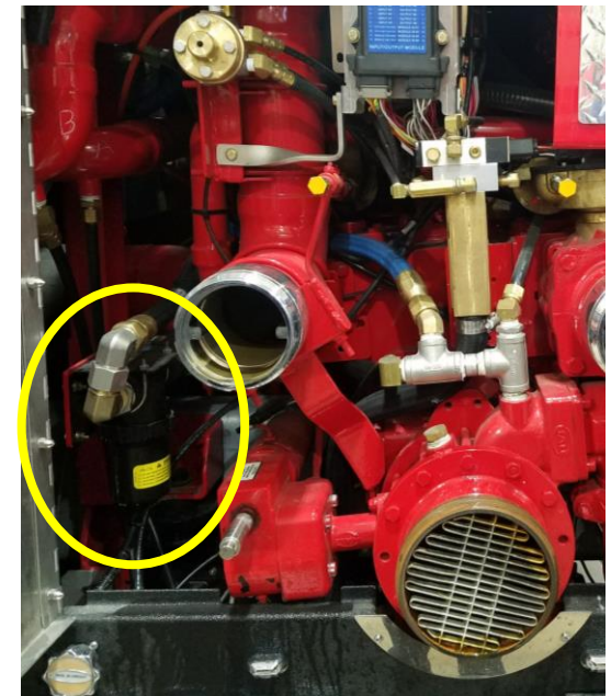
Officer side pump panel
