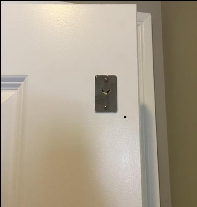
Access at top right of door
