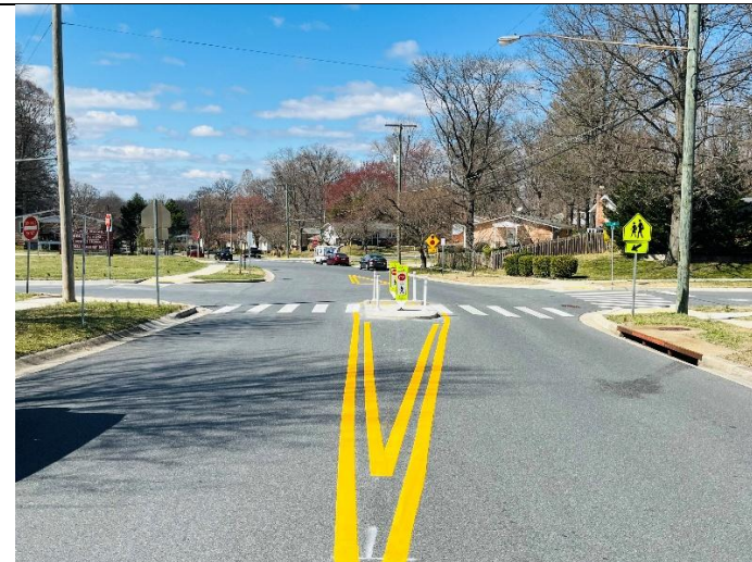
New marked crosswalk, pedestrian island, and centerline added in front of Parkland Middle School as part of building out the Safe Routes to School walkability audit recommendations.
