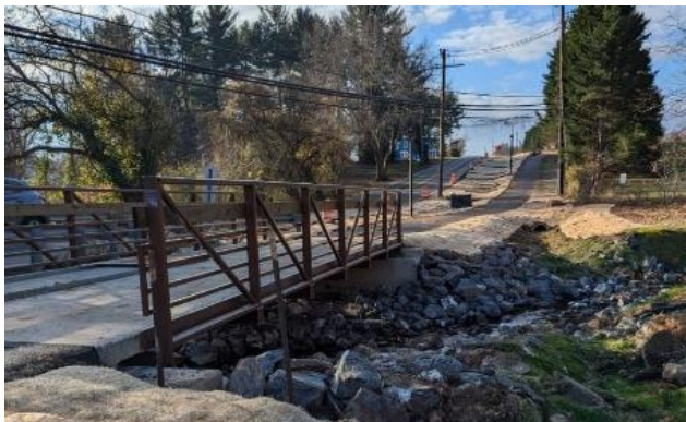
New bridge and shared use path along Good Hope Road.
