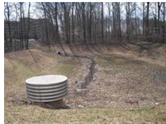
FIGURE 1. EXISTING POND (LOOKING SOUTH) TO BE EXCAVATED AT A 3:1 SLOPE. PROPOSED POND BOTTOM ELEVATION = 332.50'.
