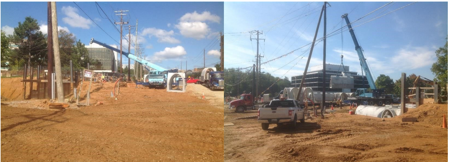
Pre-cast StormPods Installation
