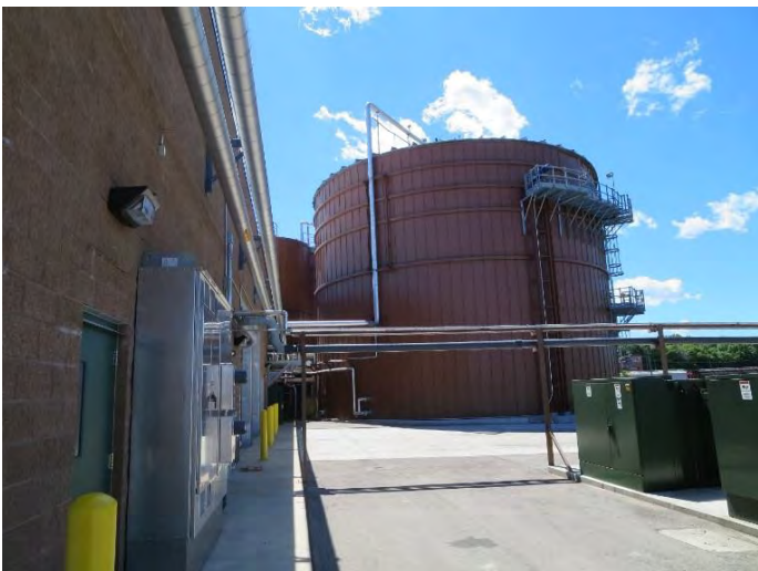
Image 3: 1.3 M gal continuously stirred tank reactor, incoming and outgoing transformers
