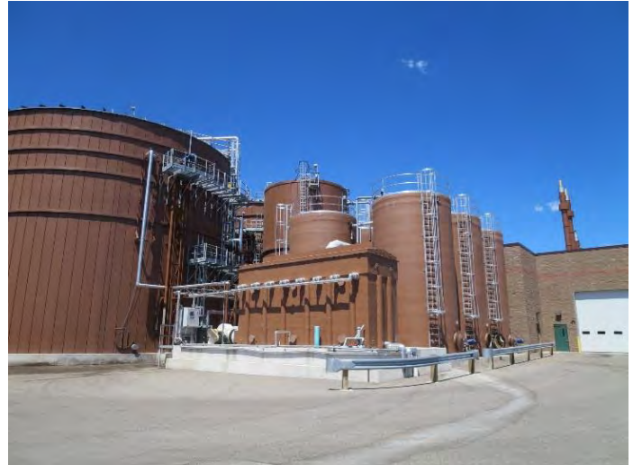
Image 2: Feedstock tank farm, biological air filter, EQ tank and digesters
